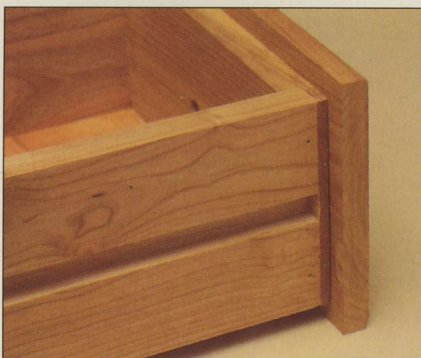
Lipped front: A rabbeted front creates a lip that serves as an overhang; useful for concealing commercial runners when the drawer is closed; lip performs double duty as drawer stop.
