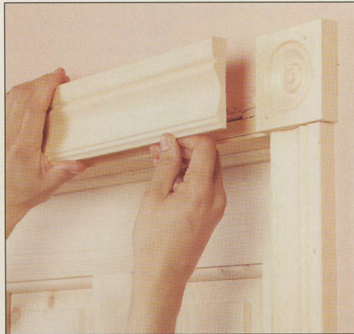
A length of head casing is fitted over a door and set against a rosette corner block. Framing a door with decorative molding serves an important esthetic function in a room.
