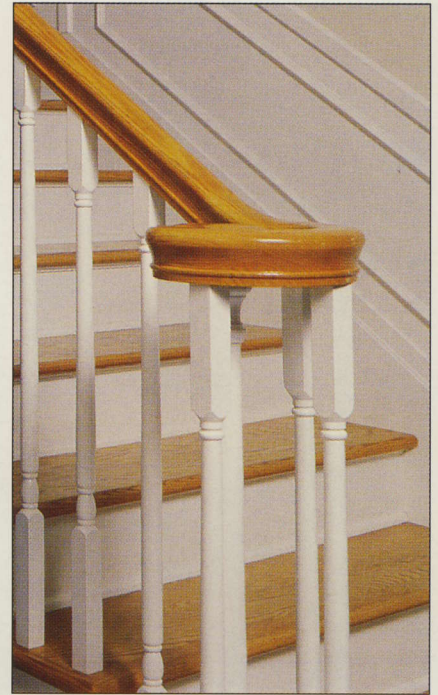
The handrail shown at right culminates in a spiral-shaped form, known as a volute, at the foot of the stairs.
