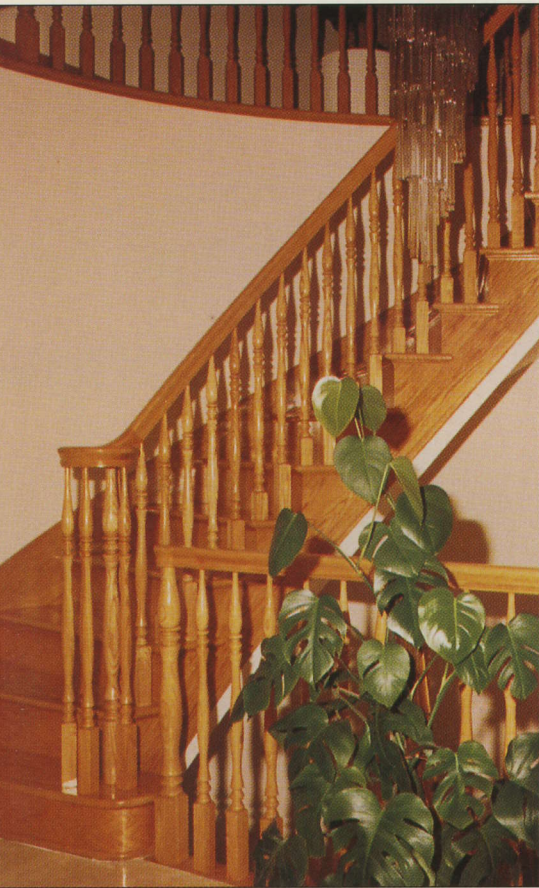
Instead of a conventional single newel post, the staircase shown above uses a series of several balusters arranged in a tight circle to serve the same visual purpose and to anchor the handrail at the base of the stairs.
