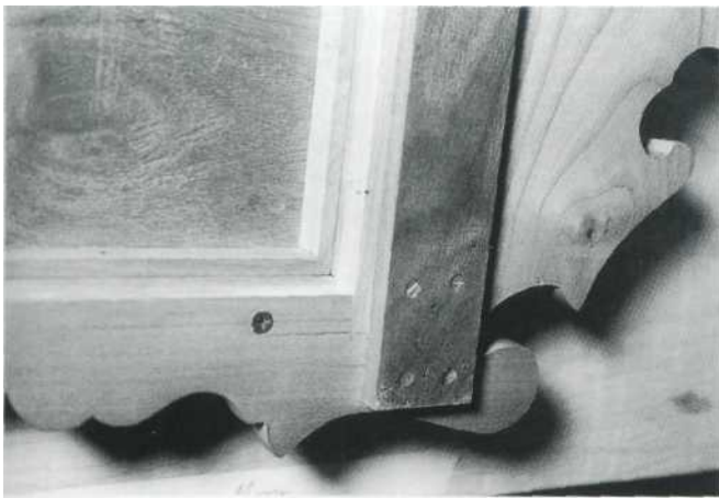
This close-up shows how the scrollwork, tack strip and cleat are assembled.
