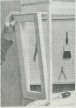
The inside edges of the panels must be rabbeted to accept the glass; they are re-moveable so that glass can easily be replaced in the event they are broken.
