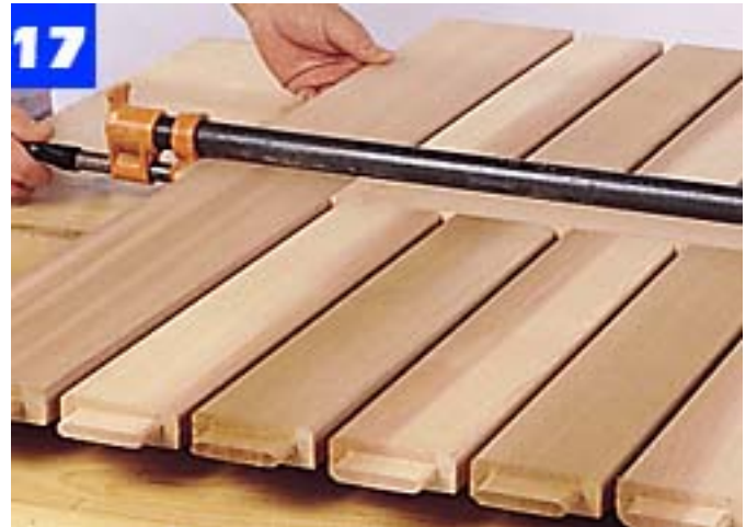
Glue and clamp a side rail to the center rail. One clamp, carefully centered, should provide enough force.
