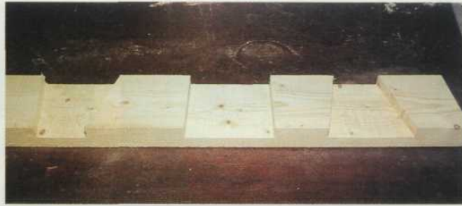
7 Detail showing dovetail pockets and the full 5" half-lap.
