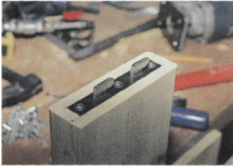
13 The knock-down hardware installed.
