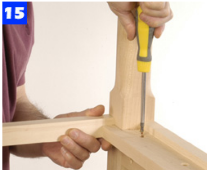
Complete the table base by joining the back subassembly to the sides and partitions. Then check for square.
