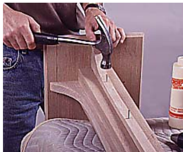
7--Attach the corbel brackets to the post sides with glue and nails. Attach them to the base with screws driven from below.
