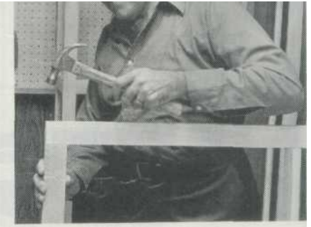
The upper, center, and lower panels are assembled with glue and nails. Pilot holes are drilled before nailing to prevent the thin wood from splitting.
