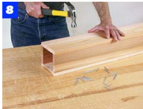
Lay out plate joints in the post parts and cut the slots. The plates keep the pieces aligned during assembly.
