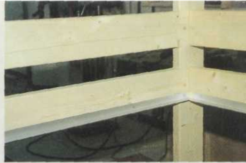
14 The aluminum "L" track is mounted 1" up from the bottom edge of the rail
