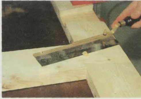
12 After the glue has dried, cut the dowels with a hand saw.
