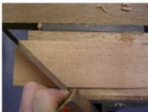
Checking both separate faces of the scarf joint from corner to corner.
