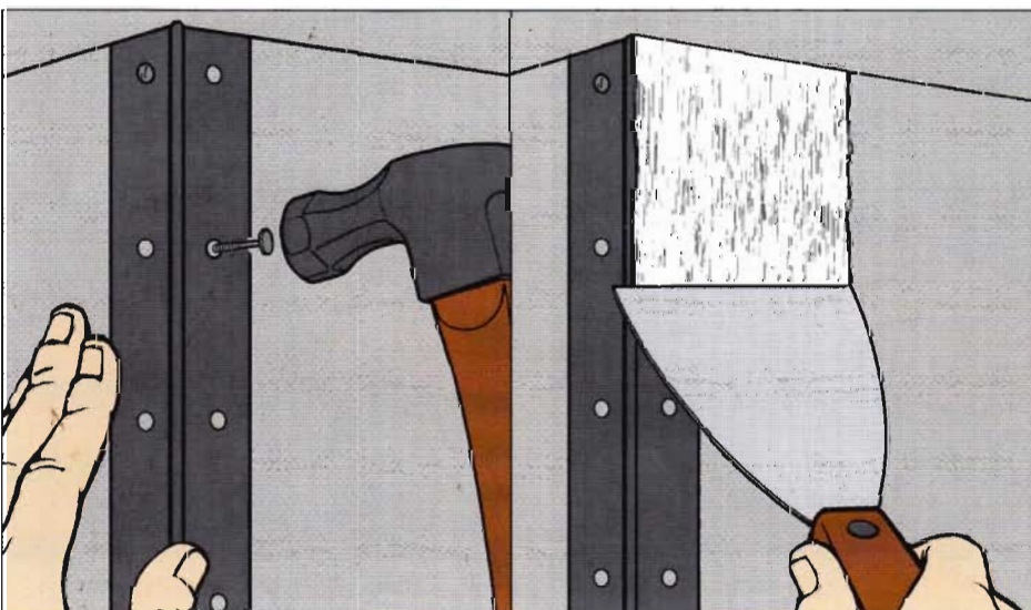
6. Nail a metal corner bead over any outside corners (left). Fill the corner with joint compound, using the raised bead edge as a guide (right).
