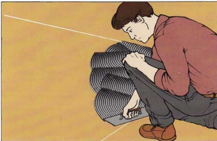
1. Spread adhesive in a relatively small area, so that you can lay the tiles before it starts to dry.
