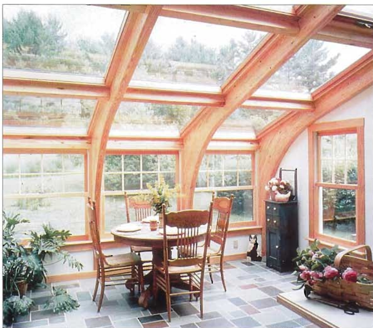
Thanks to improved glazing technology, a greenhouse addition can enhance a kitchen remodeling.
