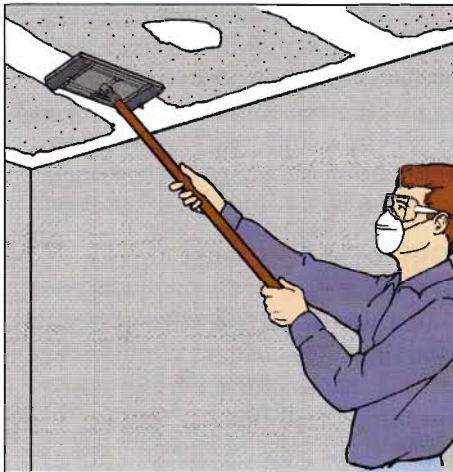
8. Sand the compound between applications. To make sanding easier, use a pole sander.
