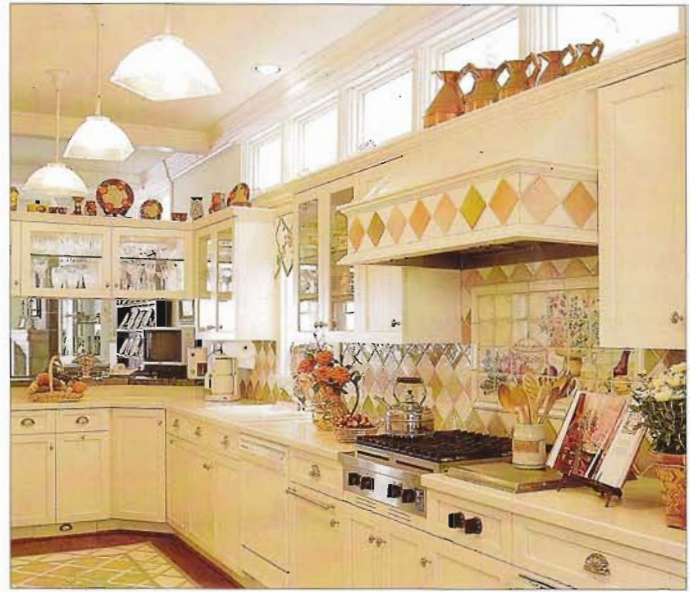
These awning windows installed into the soffit area admit light for an expansive feeling and may be opened for ventilation.
