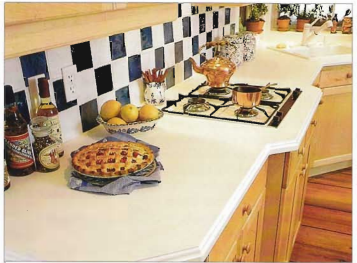
Routed edges are a special touch that's possible when you use solid-surfacing material.
