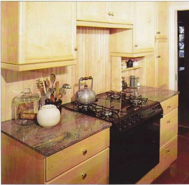
A drop-in range allows a smooth line where cabinets meet the floor, avoiding spaces that can collect dirt.
