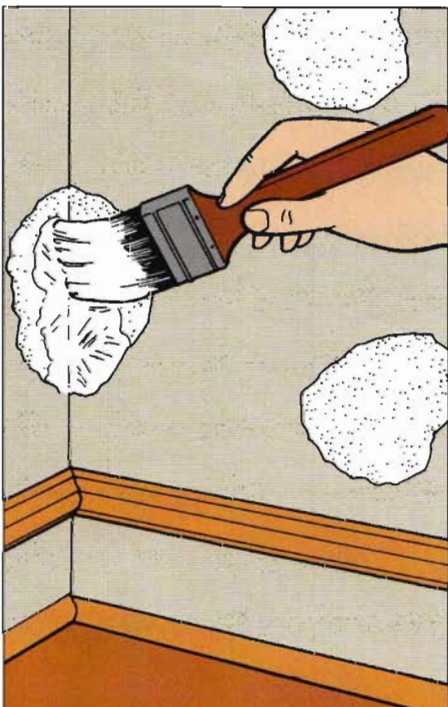
4. Spot-prime all filled areas and unpainted surfaces.
