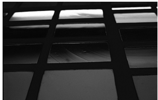
Figure 5.18 A window pane made from crown glass showing characteristic curved striations, in the window of a late seventeenth-century period room, Yale
