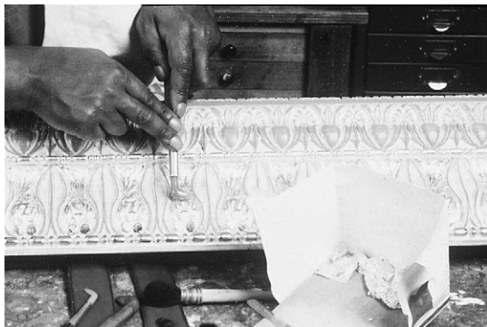
Figure 14.17 Burnishing water gilded highlights on architectural moulding using a dog's-tooth agate burnisher
