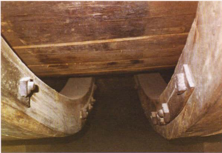
Beneath the great tun at Heidelberg, the wooden hoops, each 9 inches (23 cm) thick, hang loose.
