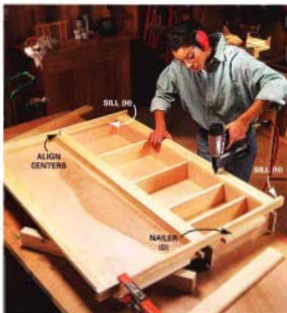
8 Center the top and bottom sills (H) and glue and nail them to the center trim. Glue and nail the side trim (G) to the sides and to the sills. Glue and nail 3/4-in. x 3/4-in. blocks to the top and bottom for nailers (D).
