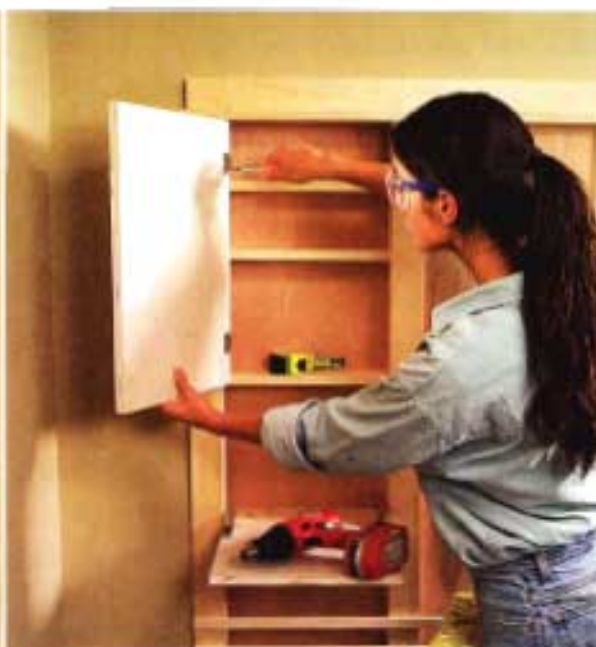
11 Screw hinges to the doors and align them in the openings. Inset doors can be fussy to adjust—use just one screw per hinge until you complete the alignment (see Handy Hint, p. 172).
