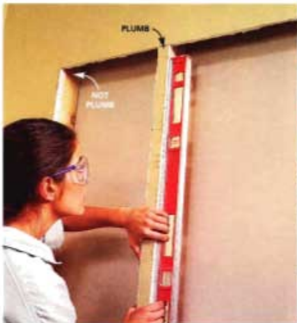
3 Check the studs for plumb and adjust the width and spacing of the boxes as needed in your plan to allow them to slip in easily (Photo 10).
