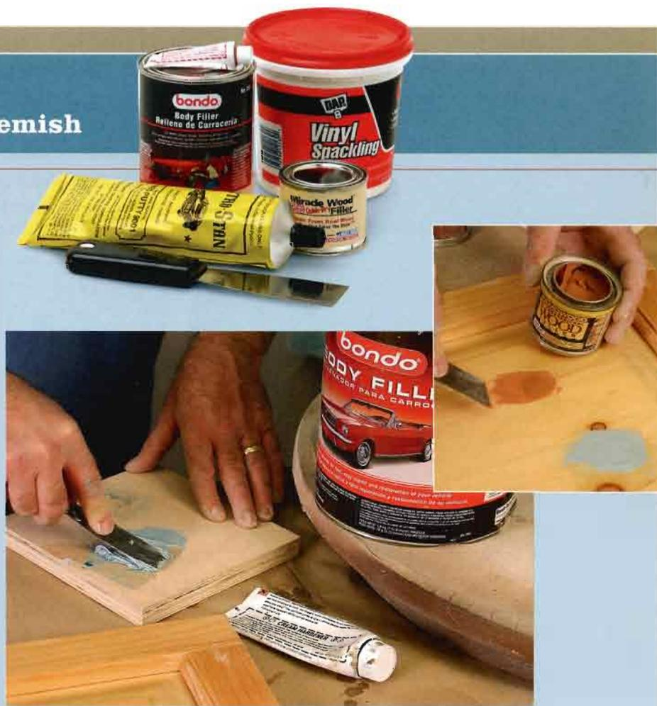
**A SMOOTH SURFACE.** Large holes are best filled with an auto-body filler that must be mixed with a hardener (above). Fast-drying wood filler is ideal for medium-size holes (center right).
