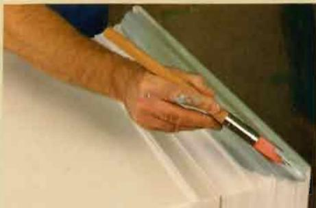
**CHOOSE THE RIGHT BRUSH.** Use a 2-in. or 2½-in. angled brush to get into small or confined areas (above). Switch to a 3-in. brush for large panels (right), and apply the paint in long, flowing strokes.
