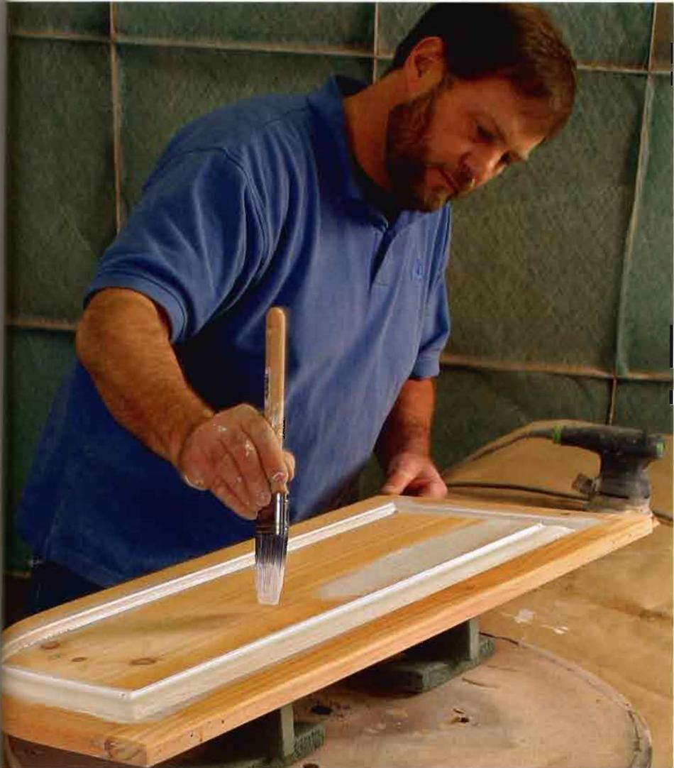
**APPLY THE FIRST COAT OF PRIMER.** Brush on an even coat. On areas that will absorb the primer, let this coat dry and then apply a second coat.
