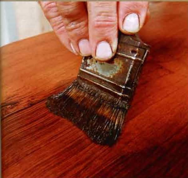
**BRUSH ON THE SECOND COAT.** A heavy coat of glaze is applied with a brush, then it's partially wiped off with the cloth pad. Less is wiped off in areas that need to be darkened.
