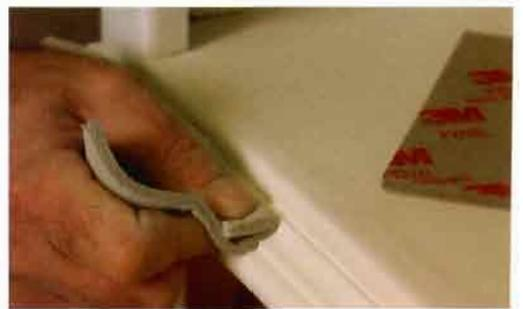
**SAND THE PRIMER.** Depending on how rough the surface is, sand the first coat of primer using P150-grit or P220-grit paper on a random-orbit sander. A sanding sponge is a good choice for smoothing moldings.
