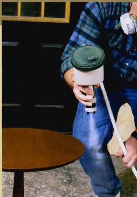
**BEGIN SPRAYING BEFORE YOU REACH THE WORKPIECE.** Hold the gun 4 in. to 6 in. away from the workpiece, and spray at a speed that makes the surface wet and shiny but not runny.
