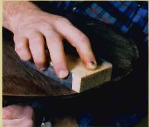
**WATERBORNE FINISHES WILL RAISE THE GRAIN.** Apply a sanding sealer over a stain or dye before any top coats. Sanding sealers contain lubricants, which make them easy to sand.
