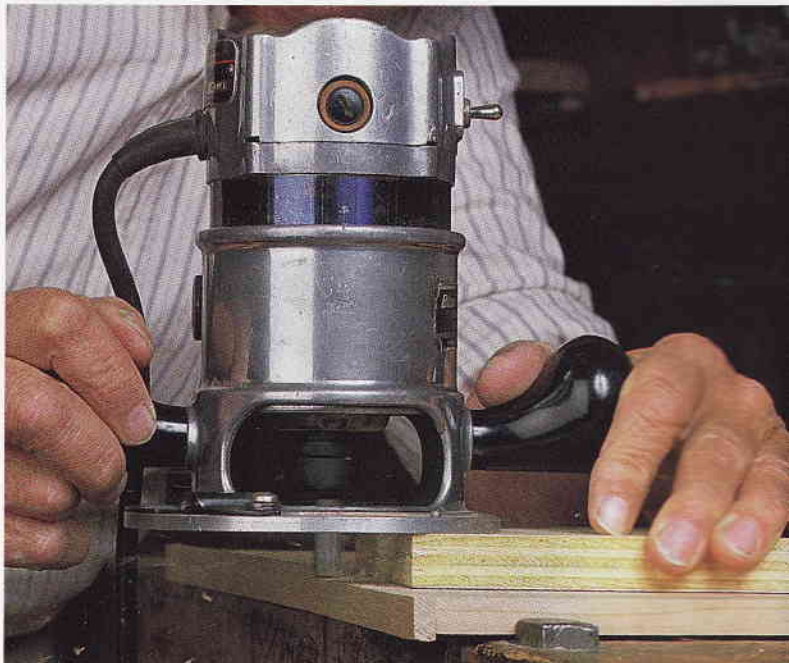
Frid guides a modified router around the table's top and bottom surfaces to flush-trim excess facing. A piece of 3/4-in. plywood is fastened to the router base and the 1/2-in.-dia. straight bit's flat end is nearly flush with the plywood base.
