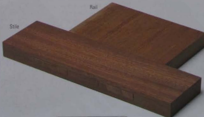
Double mortise-and-tenon joint
