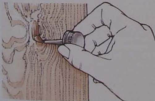
Apply two coats of knotting before priming
