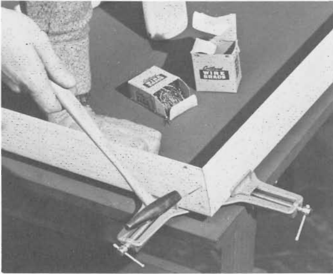
9 Clamping and nailing. With the clamshell tight in our clamp, we drive the first brad into one side near the top edge. (Don't drive the brads in all the way.)
