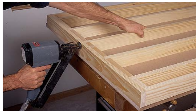
PHOTO D: With the short ribs pressed against the frame between the full-length ribs, nail or screw through the outer frame into the end of each full-length rib.
