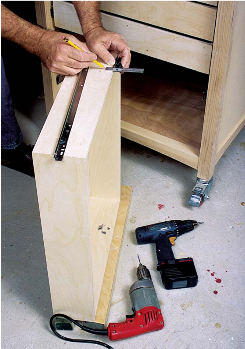
PHOTO K: A combination square gauges the lines for installing the quick-disconnect rails that attach to the drawer sides.
