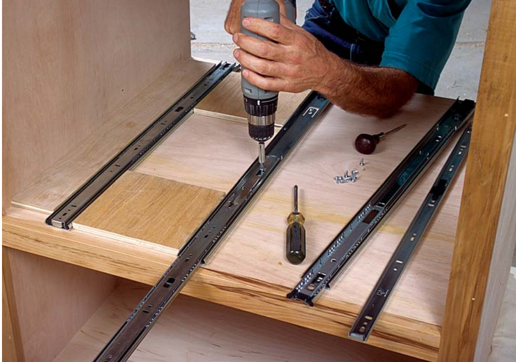
PHOTO H: After determining the drawer-slide spacing, you can make plywood spacers for easy, accurate installation of the slides.
