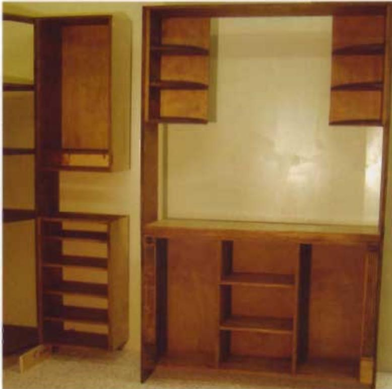
**18** I had an assistant for this installation, so I was able to assemble the center unit in my shop, then transfer it to the closet, which saved some time.
