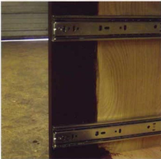
**13** These aren't deep drawers, so full extension slides were a necessity. For details on drawer slide installation, see the Shared Master Bedroom Closet project. I constructed the drawers using rabbet-and-dado joinery—this is detailed in *Beyond the Basic Box*.
