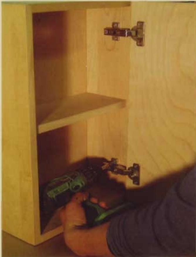
**3** With the mounting plate clicked onto the hinge cup, position the door at its correct height for mounting. I leave a  $\frac{1}{8}$ " (3mm) gap between the door and front of the cabinet (I just eyeball it, but you could tape a spacer to the edge of the door and then press it tightly into place). Using a pen, or fine marker, mark the locations of the mounting plate holes on the inside of the cabinet. A few screws will secure the door.
