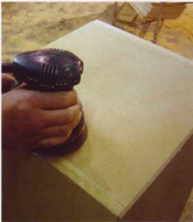
**7** When the glue has cured, remove the clamps and sand the joints flush on the top. This will be visible in the finished closet, so a smooth, uniform surface is ideal here. Any gaps can be filled with putty and resanded. I used 60- and 80-grit paper to sand down large discrepancies.
