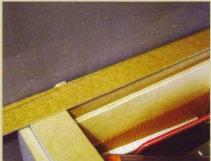
**2** Start with the back edge. Place the strip against the back wall and see how it looks: If there is no space between the strip and the wall, that will save you some time. If there is a gap, however, you'll need to scribe the strip. Set the compass points about  $\frac{1}{4}$ " (6mm) wider than the gap at its widest point. You can then run the compass along the wall and cut along the line with a jigsaw.
