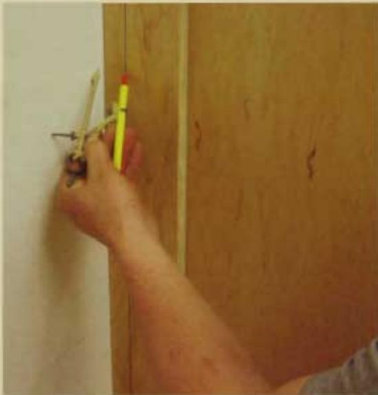
**1** Set the compass points about 1" (25mm) apart and move the compass from top to bottom to create a pencil line that mirrors the eccentricities of the wall.
