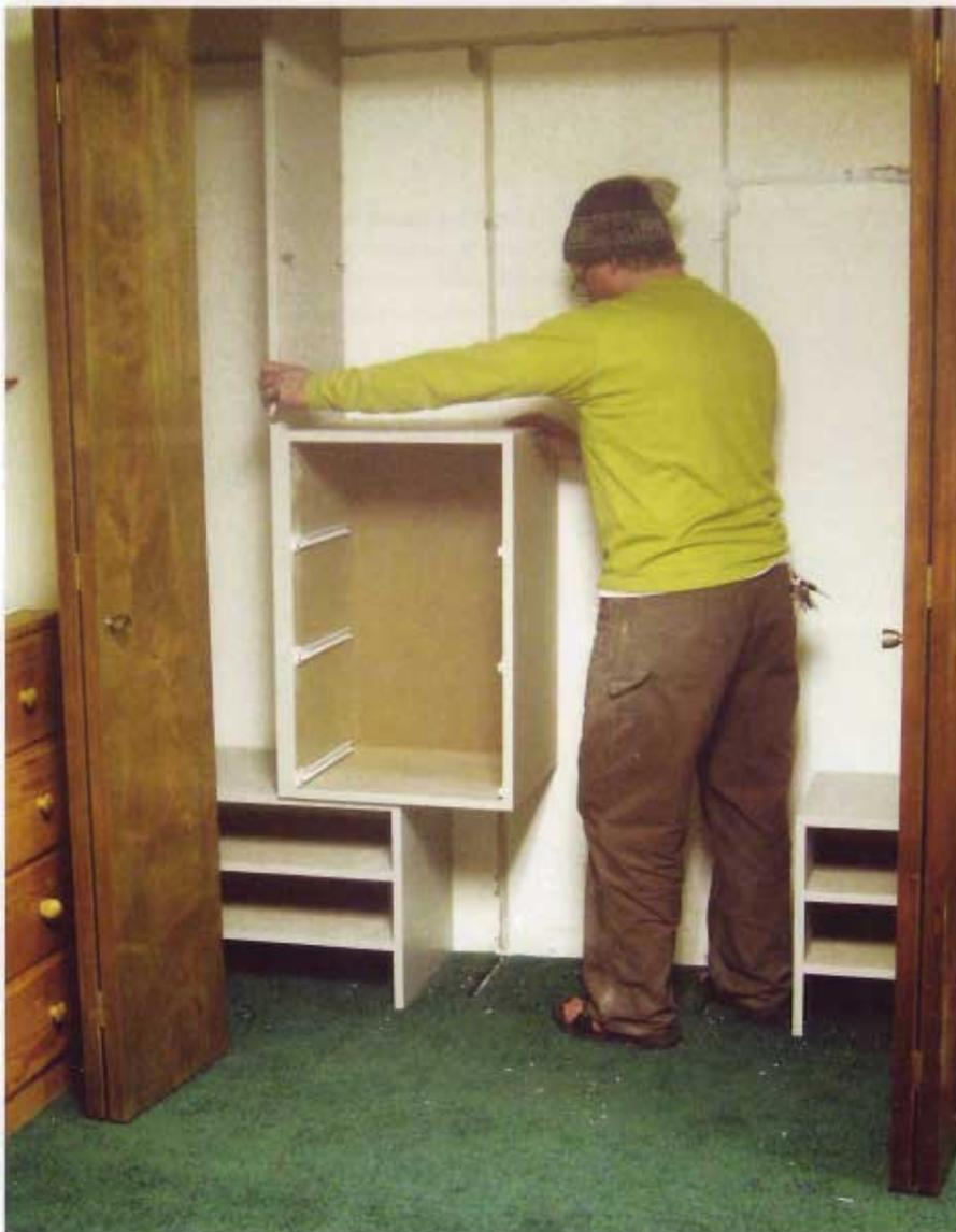
**20** Set the left-hand drawer unit in place. I kept the end panel screwed to its side to save a step, and if I had had an assistant to help me lift it, I would've kept the entire upper assembly (both drawer units and all three end panels) screwed together. That would've saved even more time.
