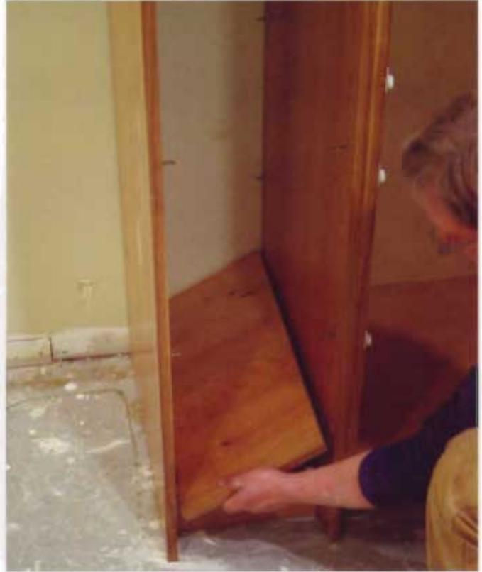
**20** The bottom shelf is placed in the tower and secured with construction adhesive.
