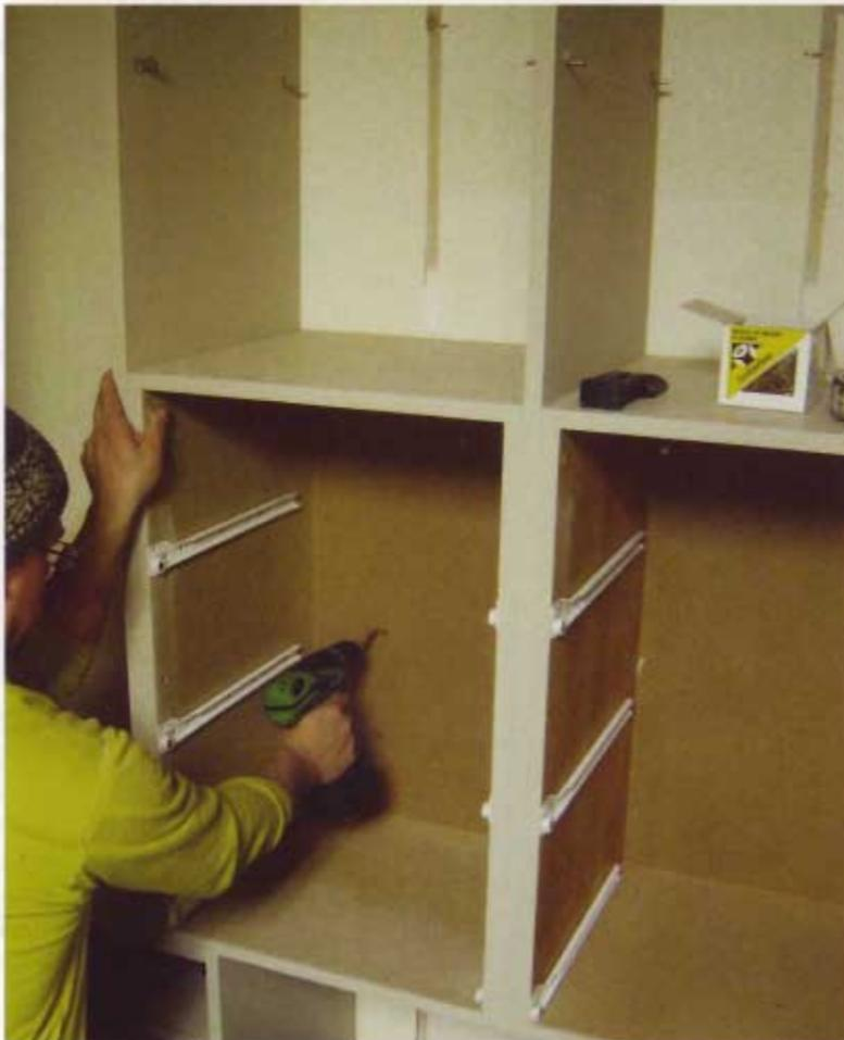
**22** Screw the drawer units into studs in the back wall. I used 12 screws, which may be more than necessary, but better safe than sorry.
