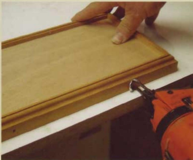
3 I attach the moulding with glue and nails.
