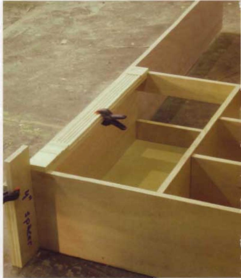
**5** The end panels are screwed directly to the cabinet. The screw heads won't show if you screw from the outside because other cabinets will cover them later. Use a 4" (102mm) spacer to position the end panels accurately.
