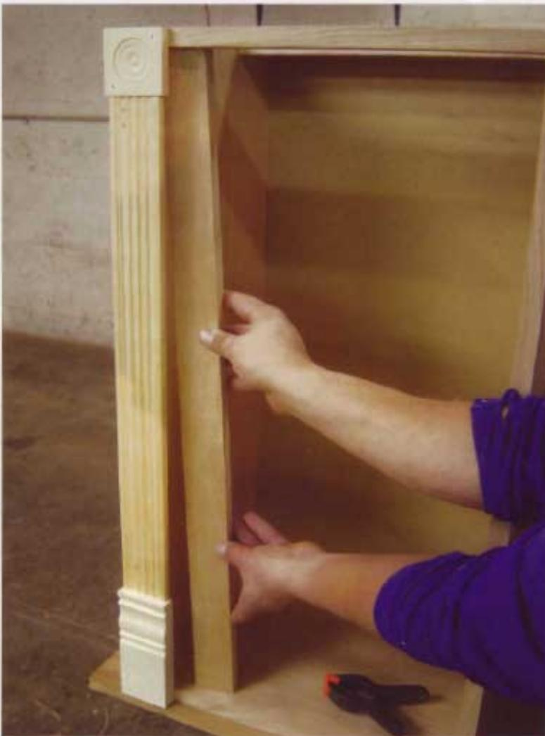
**3** You'll notice that because the trim pieces overhang in the body of the cabinet they could be easily damaged if they're not reinforced. I put in two bracing strips.
