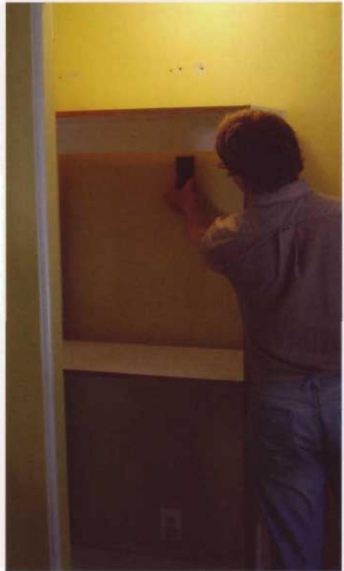
**15** Use an electronic stud finder to locate the studs in the back wall.
