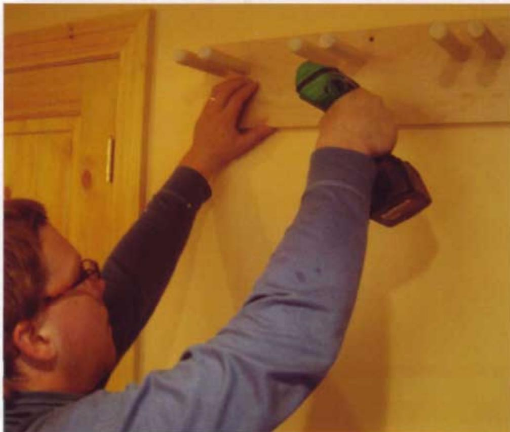
**29** Screw the ski rack into at least two studs.
