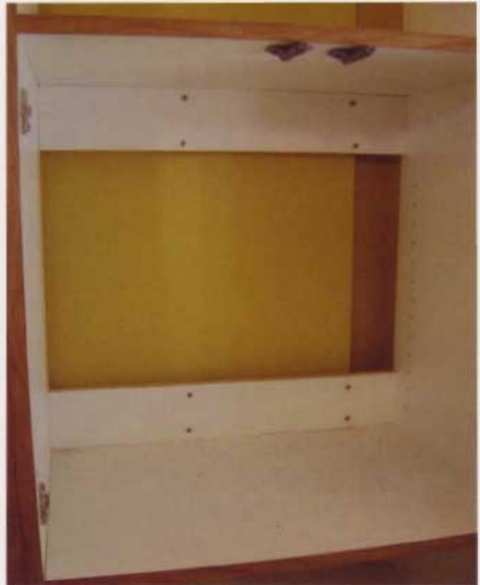
**20** Screw the smaller cabinet to the back wall, and remove the shims and temporary support.
