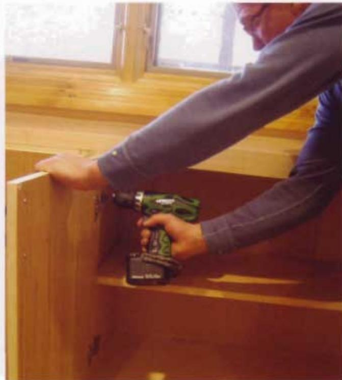
**28** Hanging the doors is straightforward. For detailed information on installing and adjusting european-style hinges, see the sidebar in the Closet-Based Home Office.
