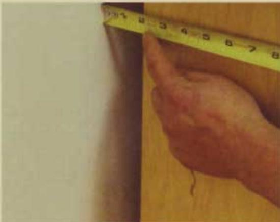
**3** To fit the filler to the gap, measure the gap at the top and bottom of the cabinet. In this case, it was about 1½" (38mm) at the top and 1" (25mm) at the bottom.
