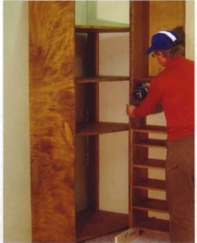
**17** The shoe cubby and the upper cabinet are screwed to the side of the corner unit. Since I took the time to mock up the installation in the shop, they are easy to align—use the screw holes to set the components exactly into place.
