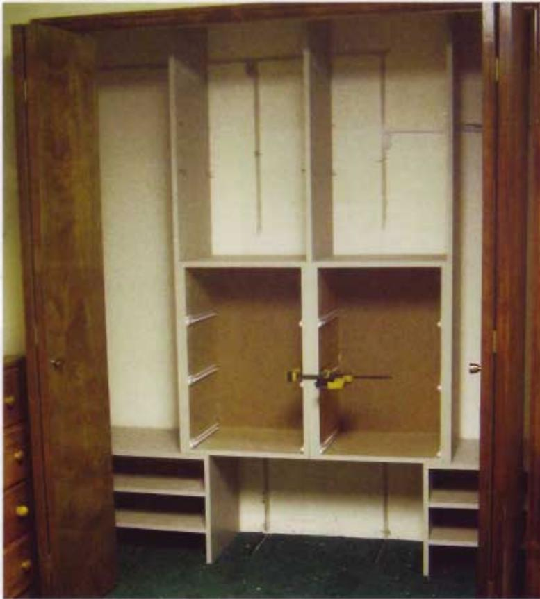
**21** The right-hand drawer unit, with end panels attached to both sides, goes in next. Align the front edges, then clamp them together with a quick-clamp. The clamp stabilizes the assembly so you can screw it together.
