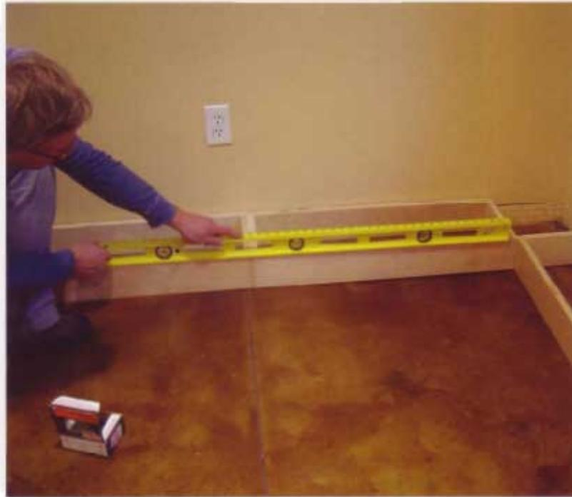
**17** I find it easier to level the bases on a long uninterrupted run like this when they are attached. Using a 4' (1219mm) level (or a laser level, if you are so equipped), locate any spots that are out of level and shim accordingly so the entire assembly of bases reads level along its entire length.
