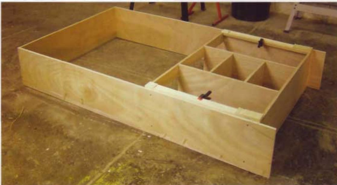
**6** The header has several functions: it serves as a place to mount the overhead lights, it provides a place to securely fasten the crown molding and it helps to create a more built-in look.
