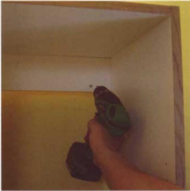
16 I recommend using two 3" (76mm) cabinet screws per stud.
