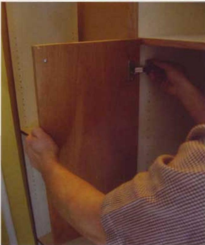
**21** The 35mm hinges make it easy to reattach the doors on site. I generally remove them while cabinets are in transit to avoid damaging them. You may need to make a couple of minor on-site adjustments to make the doors hang evenly, but it should only take a couple of minutes.
