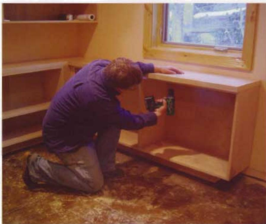
**26** The countertops are attached to the cabinets with screws from below.
