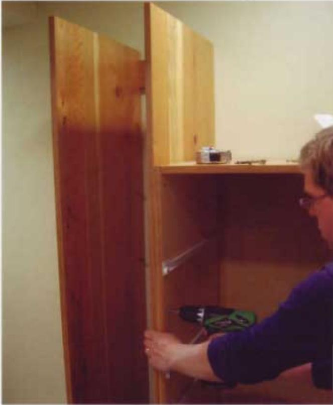
**19** Screw the tower directly to the left side of the drawer unit. It should automatically be plumb, check to make sure it is level. Shim, if necessary, and screw it to studs through its back wall stretchers.
