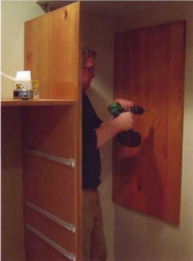
**21** Screw the short end panel into studs in the right-hand wall to create a space for the floating shelves. Place a level on top of the left-hand end panel and across the gap where the shelves will go. When the bubble is perfectly centered, mark the wall accordingly. This indicates the height at which to place the short end panel. Don't simply measure up from the floor—it could be inaccurate due to variations in the height of the flooring.
