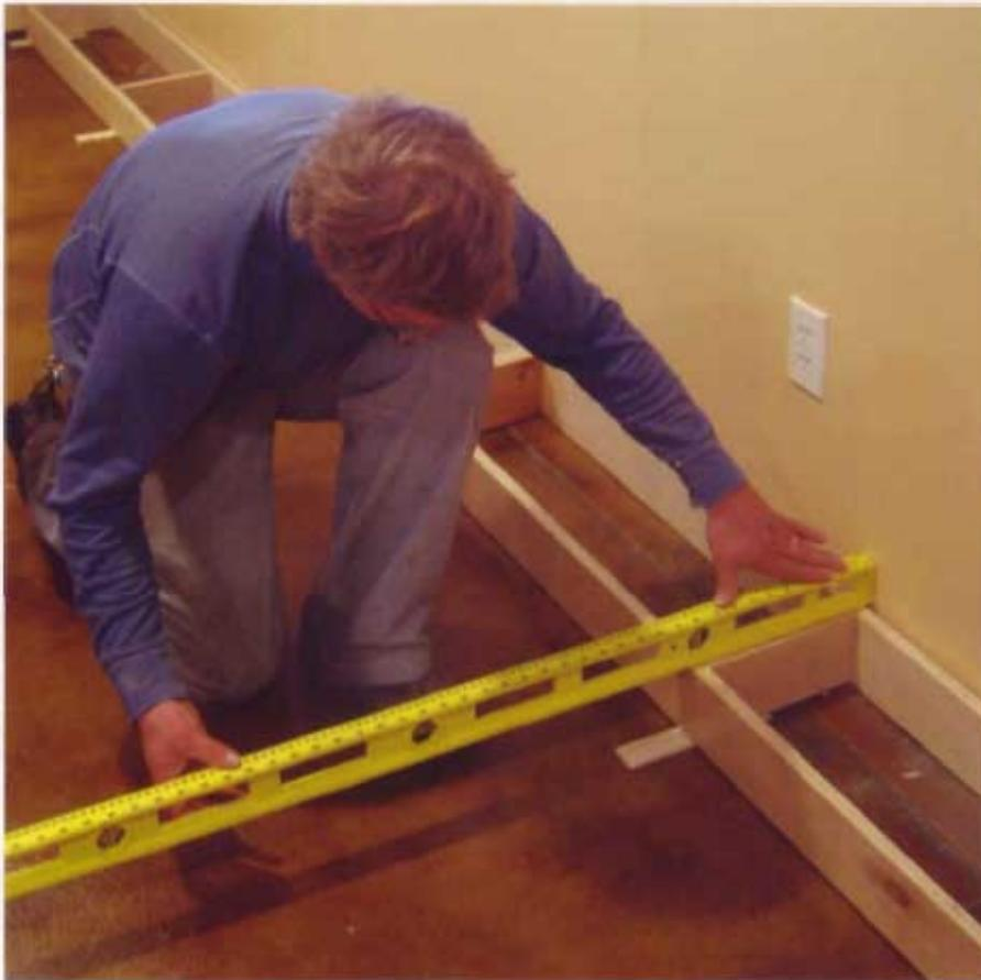
**18** Level the bases from front to back as well. Doing so makes a huge difference in how the cabinets sit against the wall.
