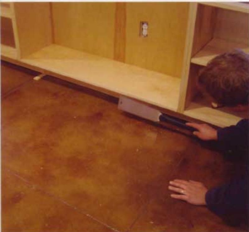
**27** Time for the finishing touches. Cut the shims flush with the cabinet bases so the toekick trim can cover them up. I used a Dozuki-style handsaw to make quick work of this.
