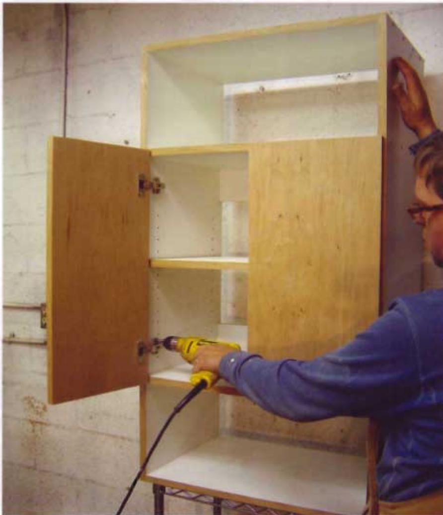
**8** Screw the hinge cups into the doors themselves, and screw the hinge plates, with the doors attached, onto the cabinet sides. With only two doors, this is an easy task.
