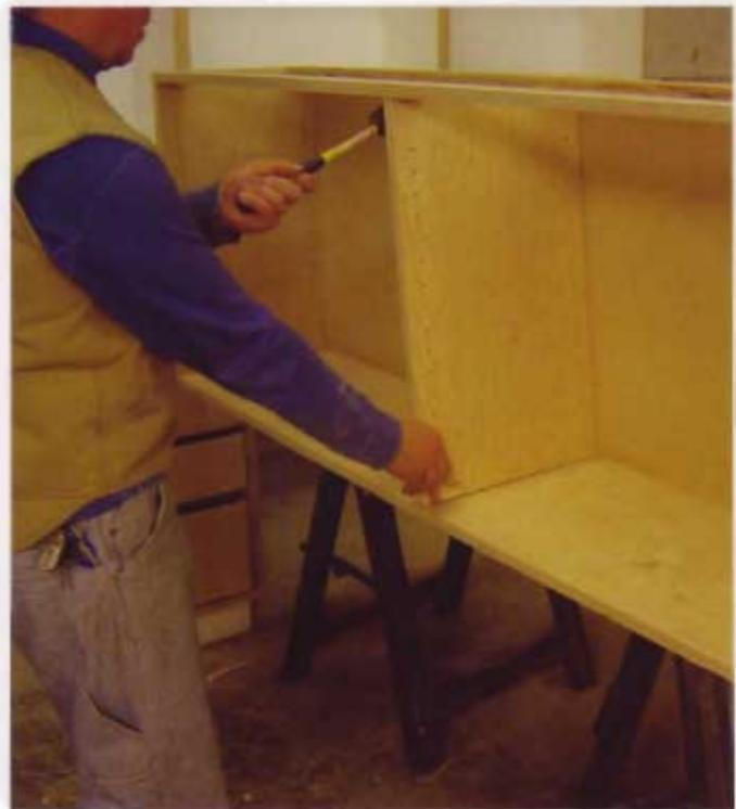
**8** Nail the partition in cabinet G through the top, bottom and back. If it is too snug, use a rubber mallet to ease it into place.
