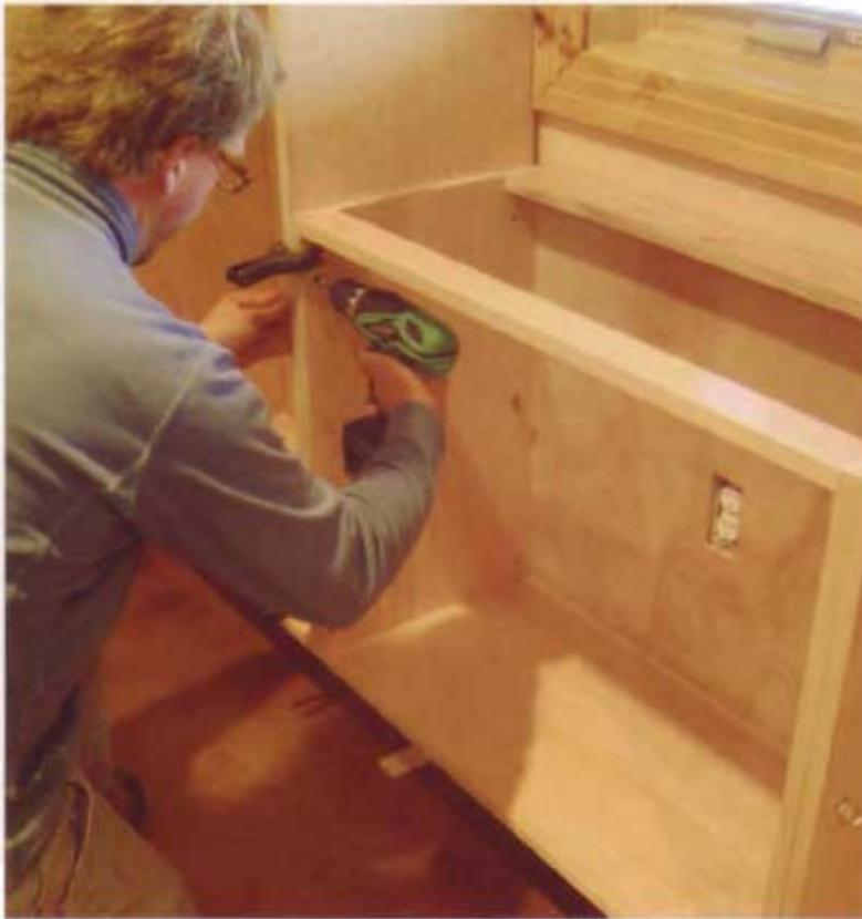
**22** Screw the cabinets together through their sides, using clamps to line up the front edges. Then screw the cabinets to studs in the wall. A stud finder will help you locate the studs behind the cabinet backs.
