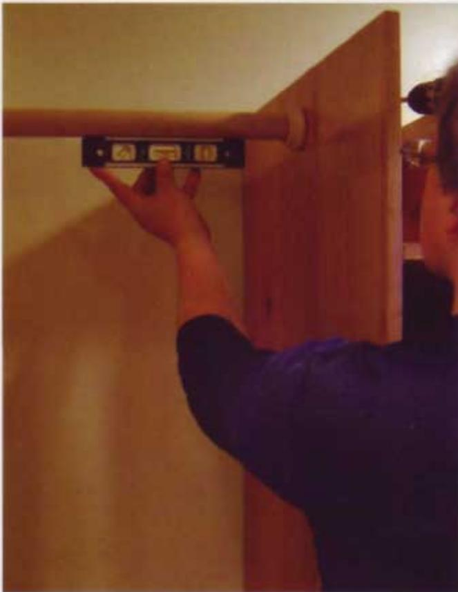
**24** Cut the clothes rods to length, then use a level to determine the correct heights for their mounting brackets. As a finishing touch, I added some crown molding, which is visible in the photo of the finished closet. For tips on installing moldings, see Beyond the Basic Box.
