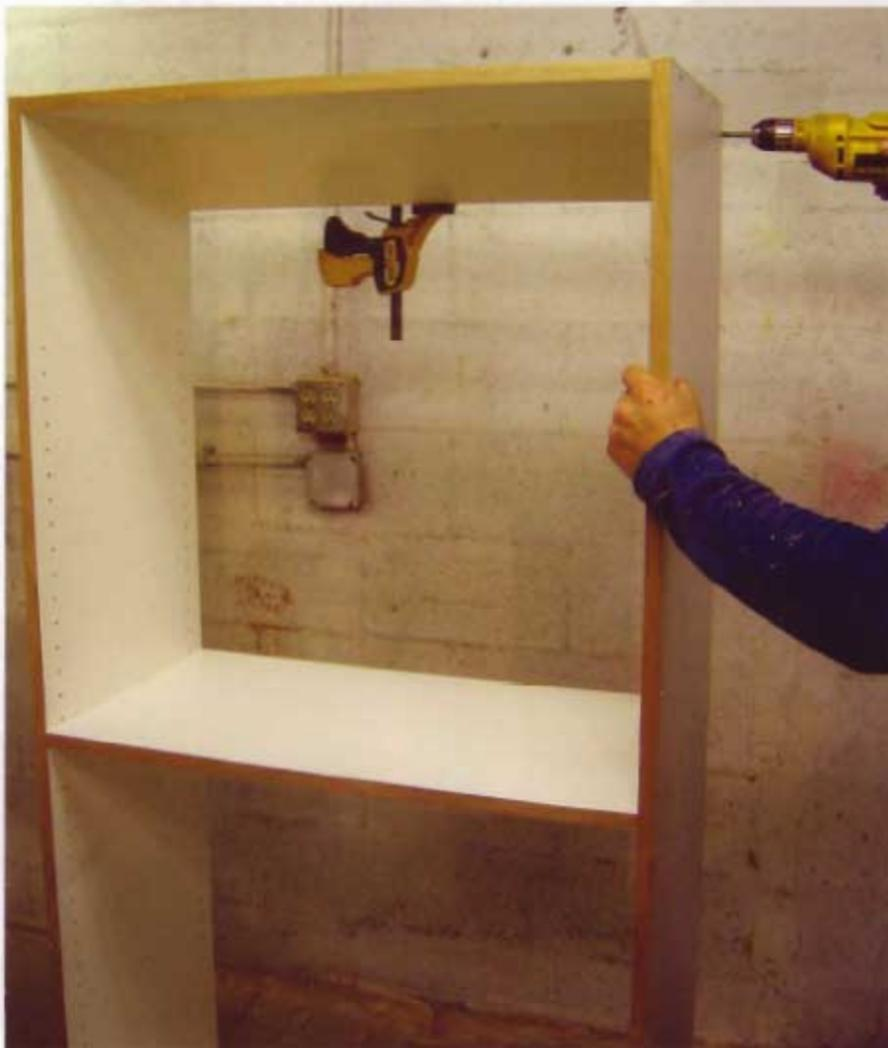
**13** Once the fixed shelf and the top have been installed, attach the back wall stretcher in place with some countersunk screws.
