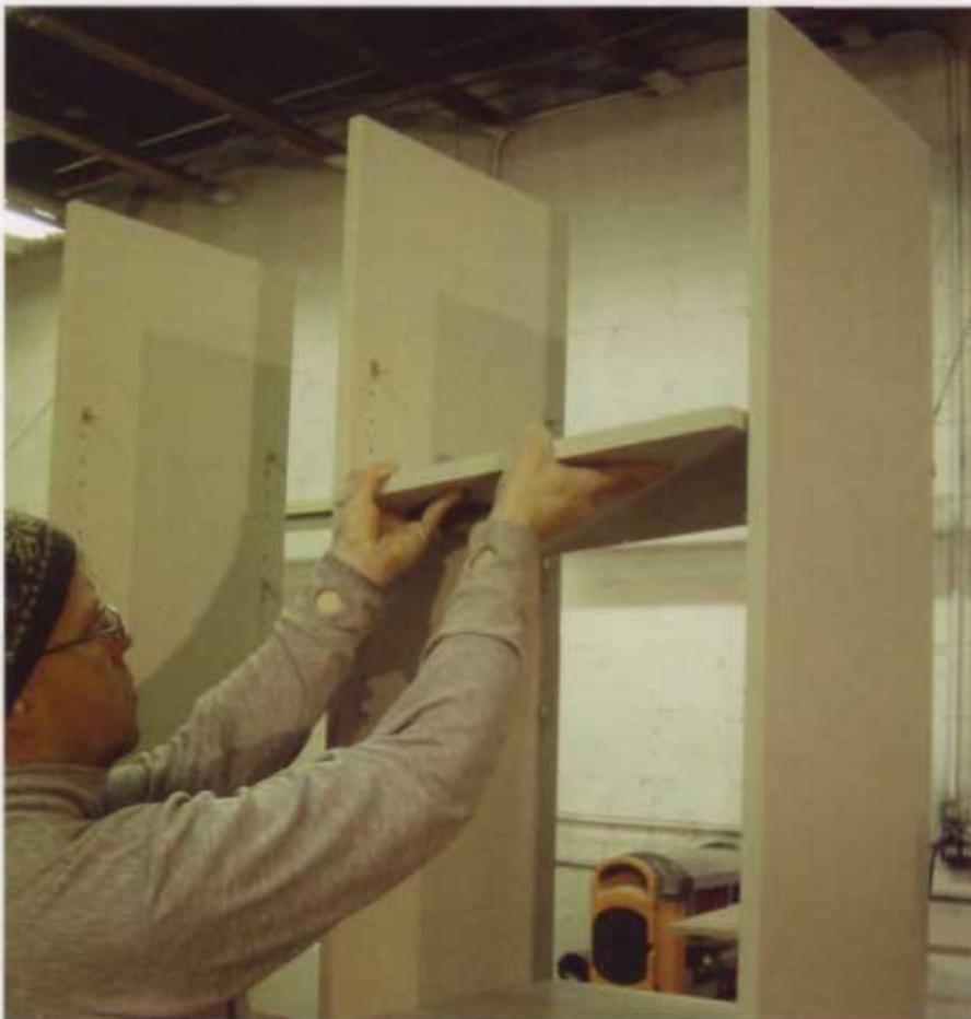
**18** You can cut and paint the MDF shelves at any time. I like to mount them on L brackets because you can run a screw through the brackets to lock the shelves in position.
