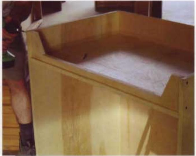
**9** The toe kick is screwed and glued into place.
