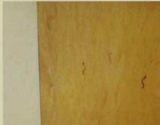
**4** I marked the filler strip accordingly [1½" (38mm) from the scribed line on the top and 1" (25mm) at the bottom], and drew a straight line to connect the two marks.
