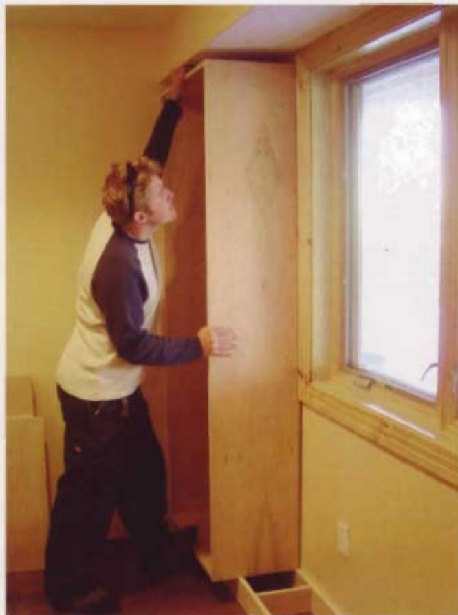
**20** To install the cabinets, start on the left-hand side of the assembly because there's a more complicated L-shape grouping on the right-hand side which will require the use of a filler. The cabinets at the left are positioned flush against the wall.
