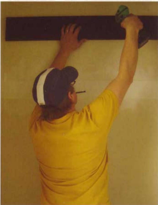
**15** This installation was easy. I removed the old shelf and coat rod first (note the primer on the wall where they used to be). Once the primer dried, I touched up the paint to conceal all traces of the old unit. Then I screwed the back wall cleat to studs.
