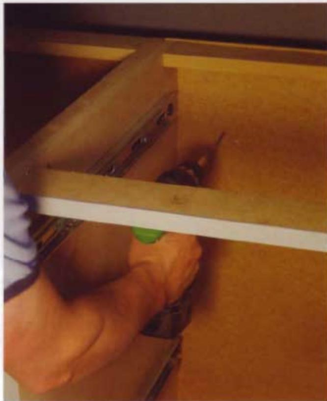
11 I screwed the cabinets into studs in the back wall.
