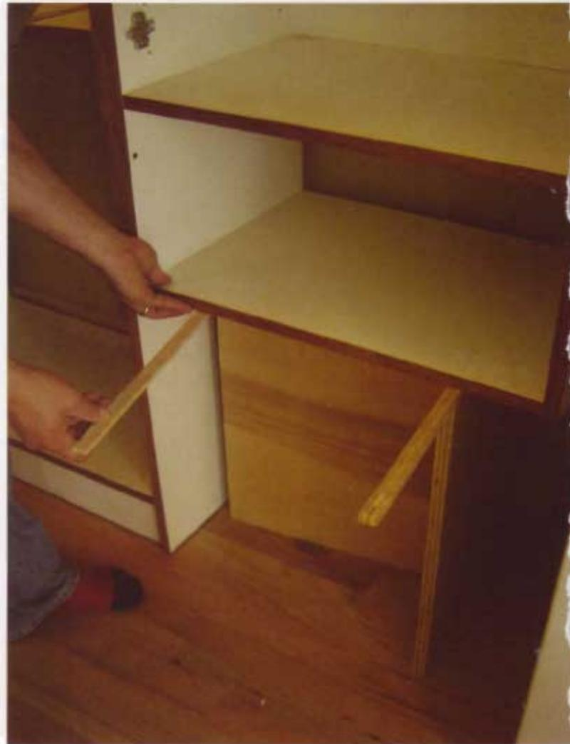
18 For some wiggle room, build the temporary support  $\frac{1}{4}$ " (6mm) shorter than the finished height. I used shims to align the top edges of the cabinets.
