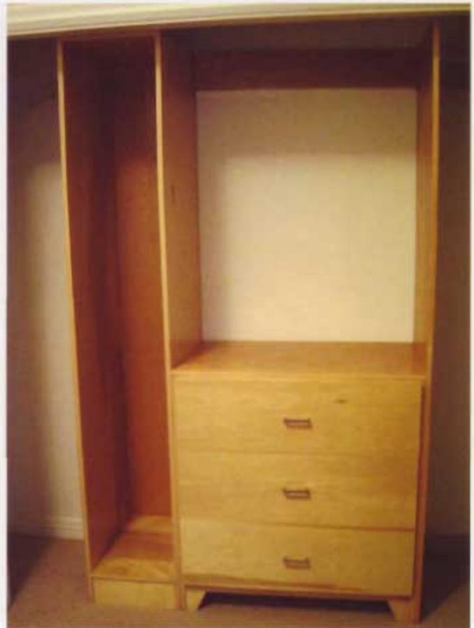
**14** By setting up the components in the shop beforehand, I can rest assured the installation will go smoothly. Because this design is pretty simple, I'll just have to screw the components to the wall and install the clothes rods.
