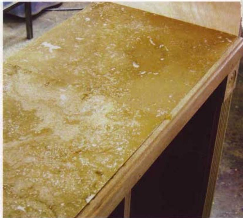
**11** I tested the fit of the tiles and I needed to remove about  $\frac{1}{16}$ " (2mm) from the edges. A quick pass over my stationary belt sander shaved it off and created a perfect fit. I waited until the rest of the project was stained and varnished before laying the tiles with construction adhesive. I coated them with stone sealer per the manufacturer's directions.
