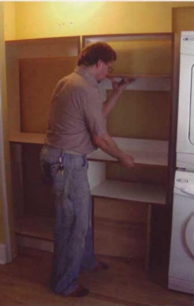
17 Since I performed the installation by myself, I built a temporary stand for the wall-hung cabinet. It consists of two plywood scraps that I nailed together in the shape of a T, and it provided all the support necessary to keep the cabinet in place while I fastened it to the wall.
