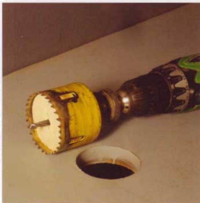
**14** For ease of cable management, I drilled a 2½"-diameter (64mm) hole through the desktop near its back edge. I trimmed out the hole with a brushed nickel grommet.
