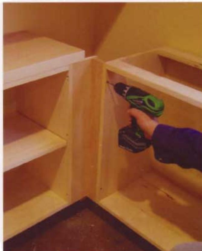
**25** Attached the narrow filler to cabinet G, which is also screwed through the back side of the filler that is attached to cabinet F.
