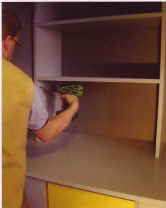
**13** Set the bookcase directly on top of the desktop and screw it to the wall through its left-hand side.
