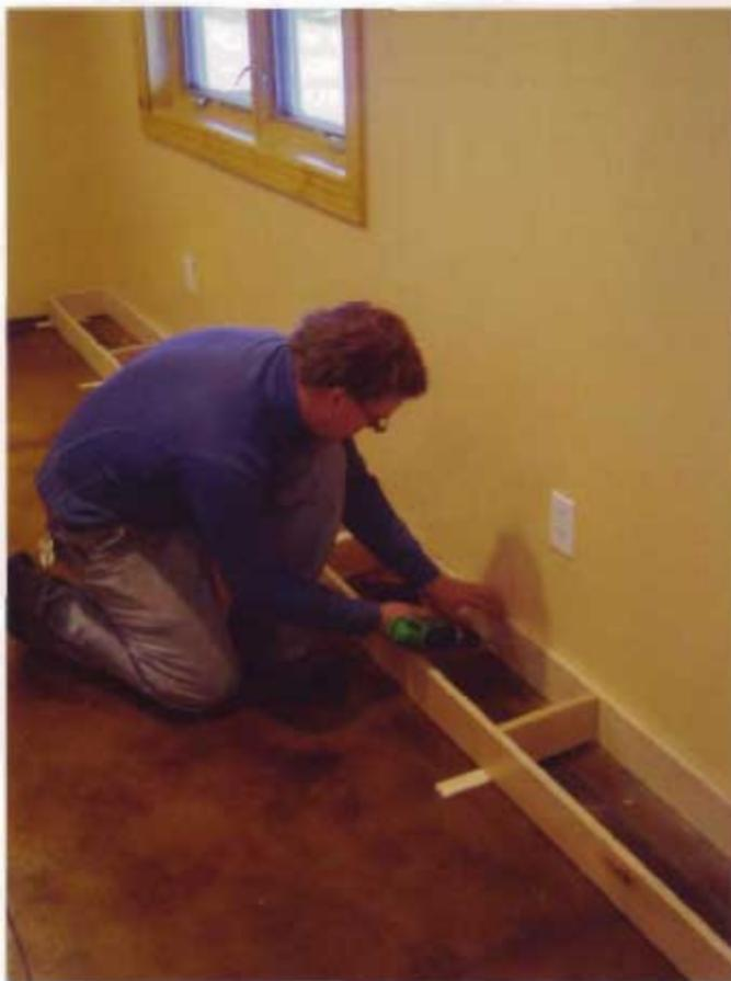
**19** Screw the bases into studs in the back wall so they won't move around when you set the cabinets.
