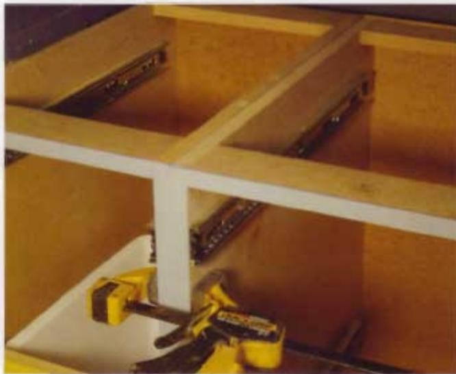
10 Once you've set the base into position and leveled it with shims as needed, you can set the cabinets on it. I pushed the cabinets up against the right-hand wall, then screwed them together. You'll notice that I used a quick-clamp to keep their front edges flush. This configuration left an uneven gap along the left-hand side due to some bulges in the plaster on the wall. I scribed a filler strip to fit this space.
