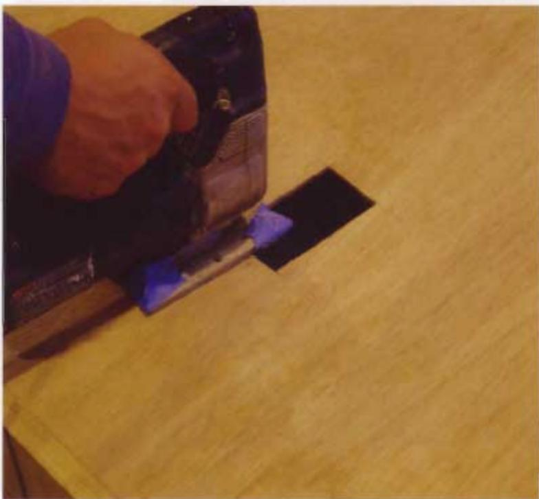
**21** Cut holes into the cabinet backs where needed for electrical outlets. A jigsaw does the job quickly and neatly.
