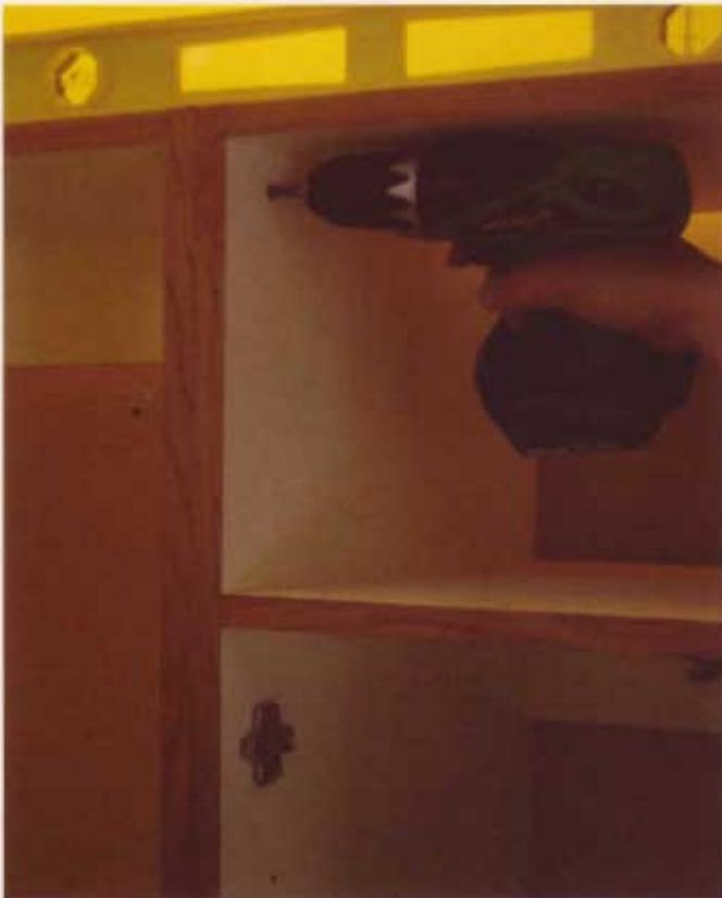
**19** Once the front edges of the cabinets are screwed together with 1<sup>1</sup>/<sub>4</sub>" (32mm) self-tapping screws, the separate units will start to read as one unit. If you took the time to mock up the installation in the shop, as I did, the screw holes will already be in the right places and this step will be a snap. Either way, I suggest using a quick-clamp to hold the edges flush while you're putting in the screws.
