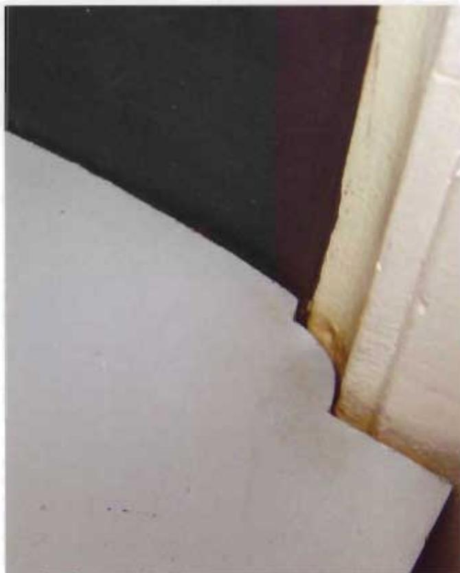
**12** In a perfect world, the closet niche would be a precise rectangle, and you could just measure it and cut a rectangle to fit for the desktop. If you're lucky and this is the case, go for it! Otherwise, I suggest using a method for creating a template that will help you to fit a desktop or work surface into an uneven spot. (This also works great for countertops, by the way.) See the sidebar on page 62.
