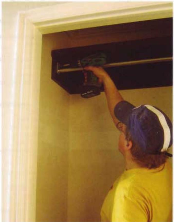
**16** I next screwed the side wall cleats into studs. Once I dropped the shelf into place and screwed in the coat rod, I vacuumed the closet and set the cabinet into place.
