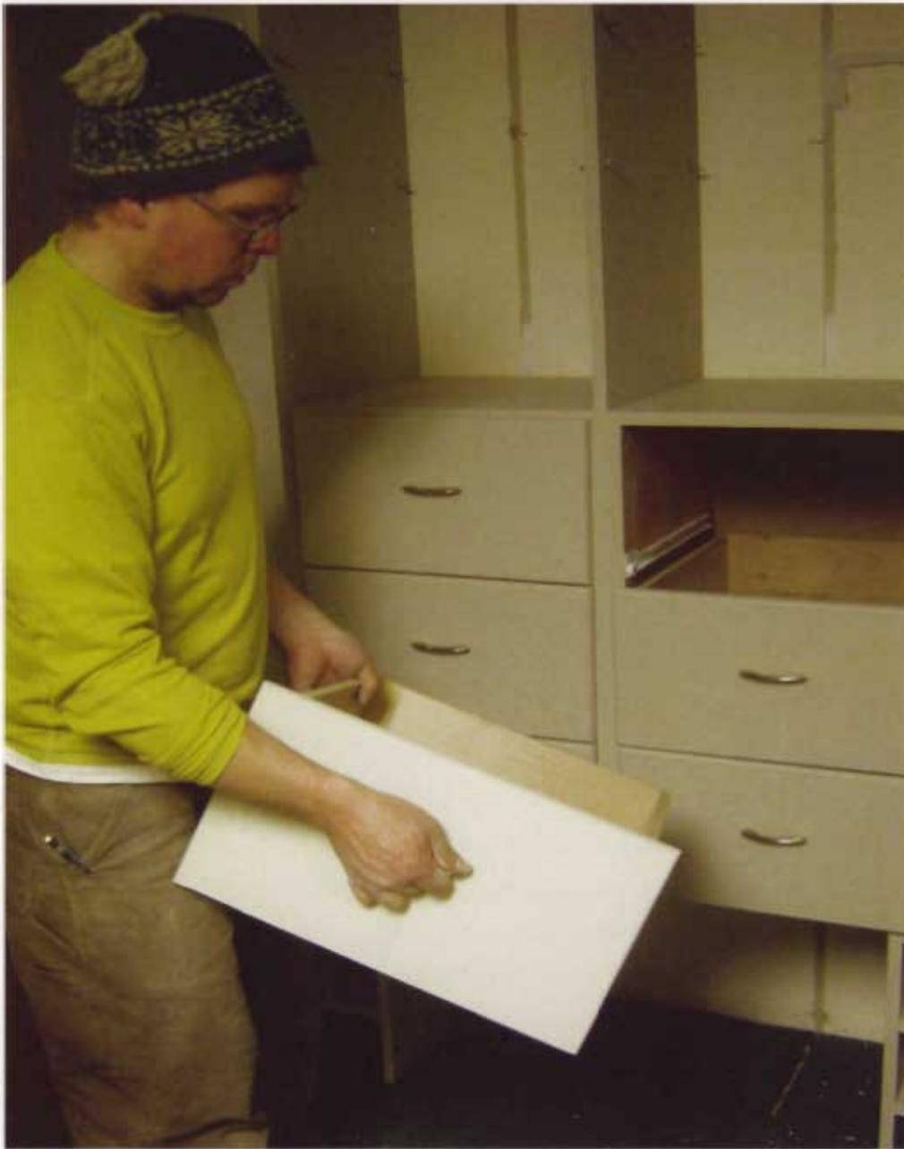
**23** Prior to loading the parts in the van, I removed the drawers from the preassembled installation. As I removed them, I labeled them according to their position in the finished unit—it would be easy to get them mixed up otherwise. The clothes rods were easy to install. For the drywall anchors, I used 3" (76mm) toggle bolts because there weren't any studs where I needed them.
