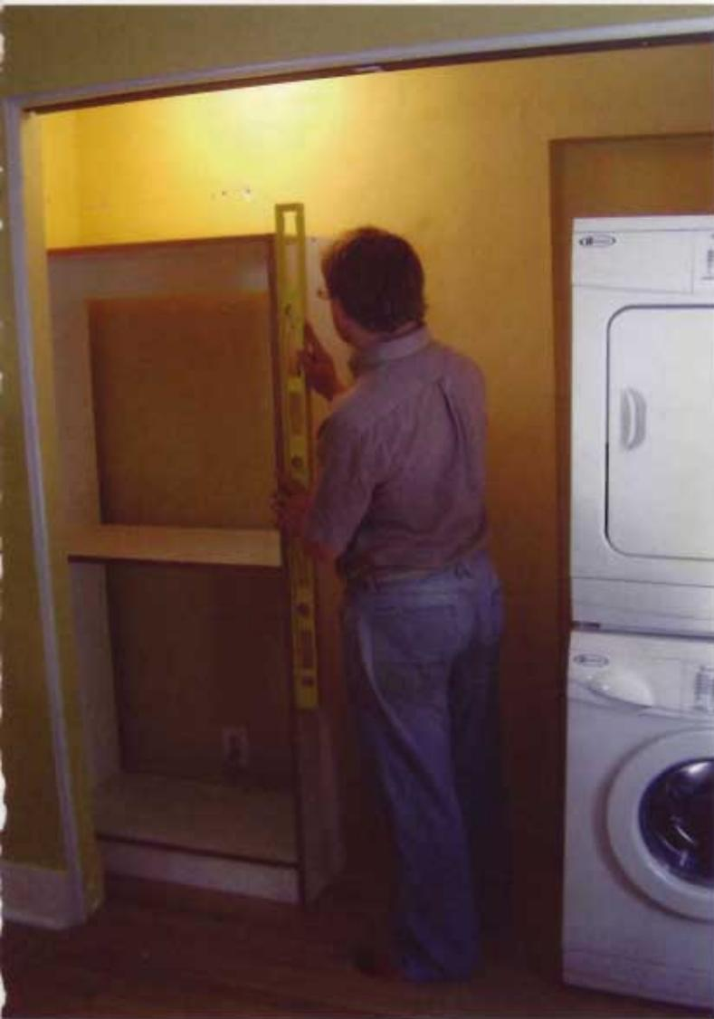
**14** After clearing out the closet niche, I installed the large cabinet first. Use a 48" (1219mm) level to determine whether you need to shim the cabinet to make it plumb and level.
