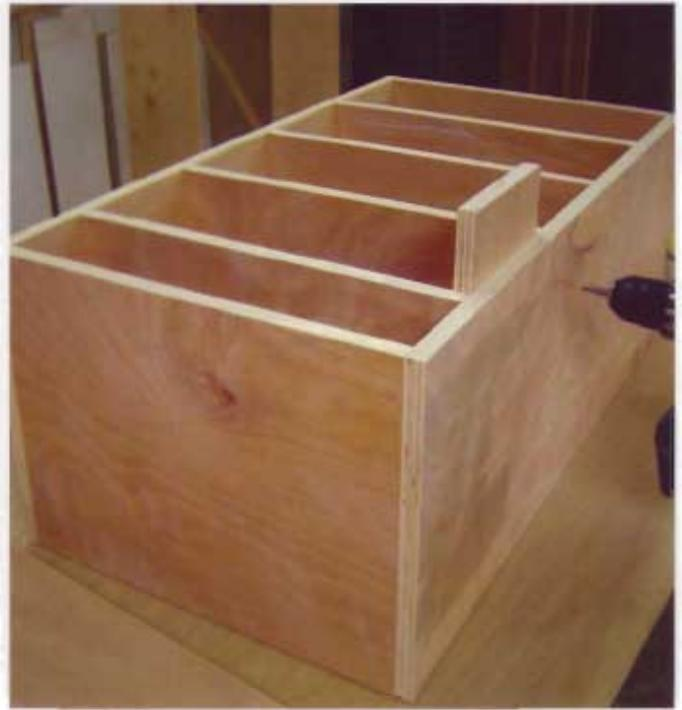
**14** To assure uniform spacing of the shoe cubbies, use a 5" (127mm) spacer. The highest shelf is slightly shorter.
