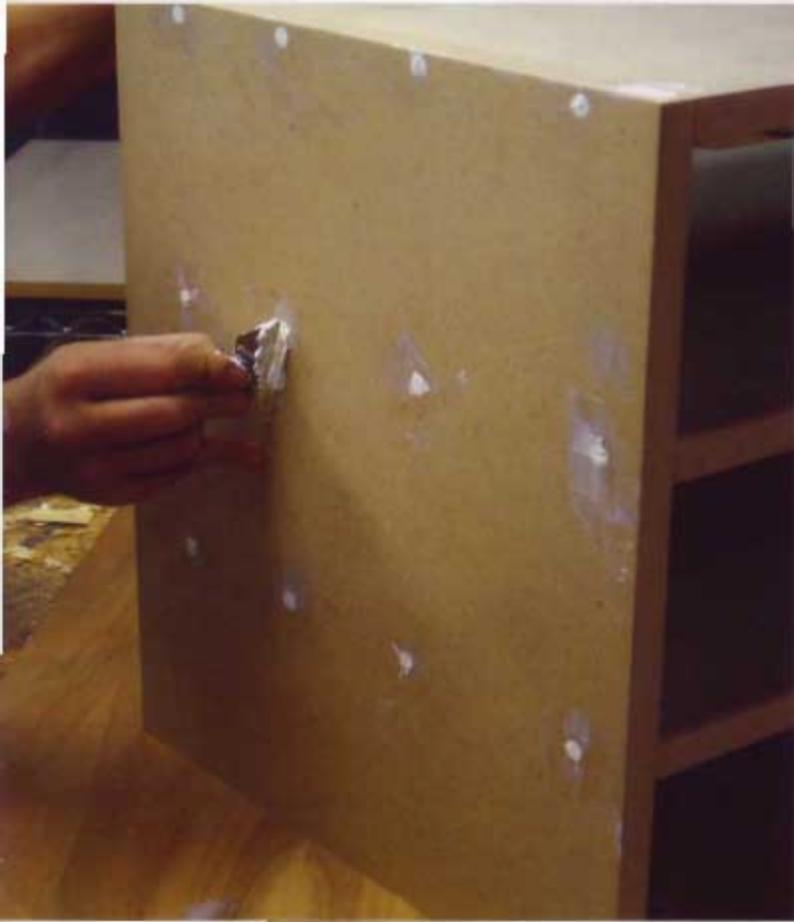
**10** Fill all visible screw holes with a non-shrinking putty, then paint.
