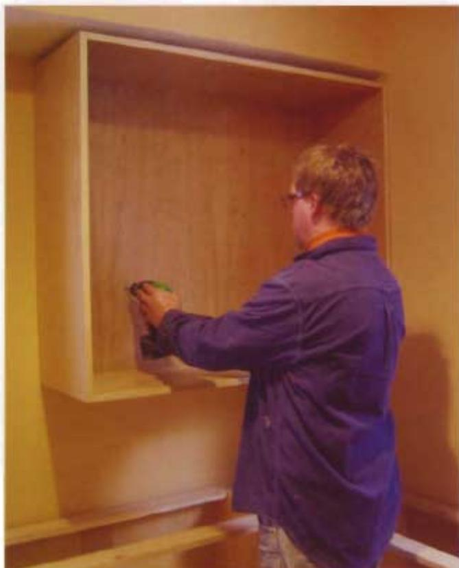
**24** Screw the wall cabinet to the wall in six places. If you're working alone, you can prop up the cabinet on a milk crate and use some scrap wood to lift it to the right height.
