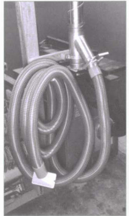
Adding a vacuum hose to your collection system makes shop cleanup quick and easy. This 2½-in. flexible hose, controlled by its own blast gate, connects via a lateral tee to ductwork servicing a stationary machine.
