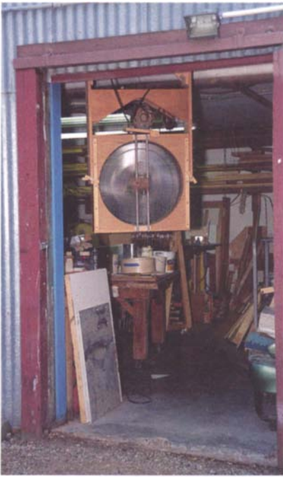
Roger Heitzman's clever shopmade ventilator, mounted in front of his shop's sliding door, uses a high-speed exhaust fan to blow dusty air out of the shop. The device swivels up and out of the way when not in use.
