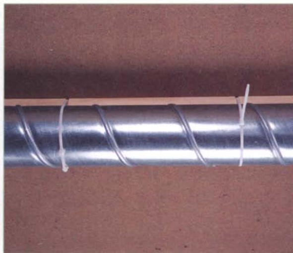
A convenient way to install ductwork atop a paneled or dry-walled surface is to use 1x2 strips nailed or screwed along the path of the duct. The duct mounts atop the strips, which are grooved to allow fastening with self-locking plastic ties.
