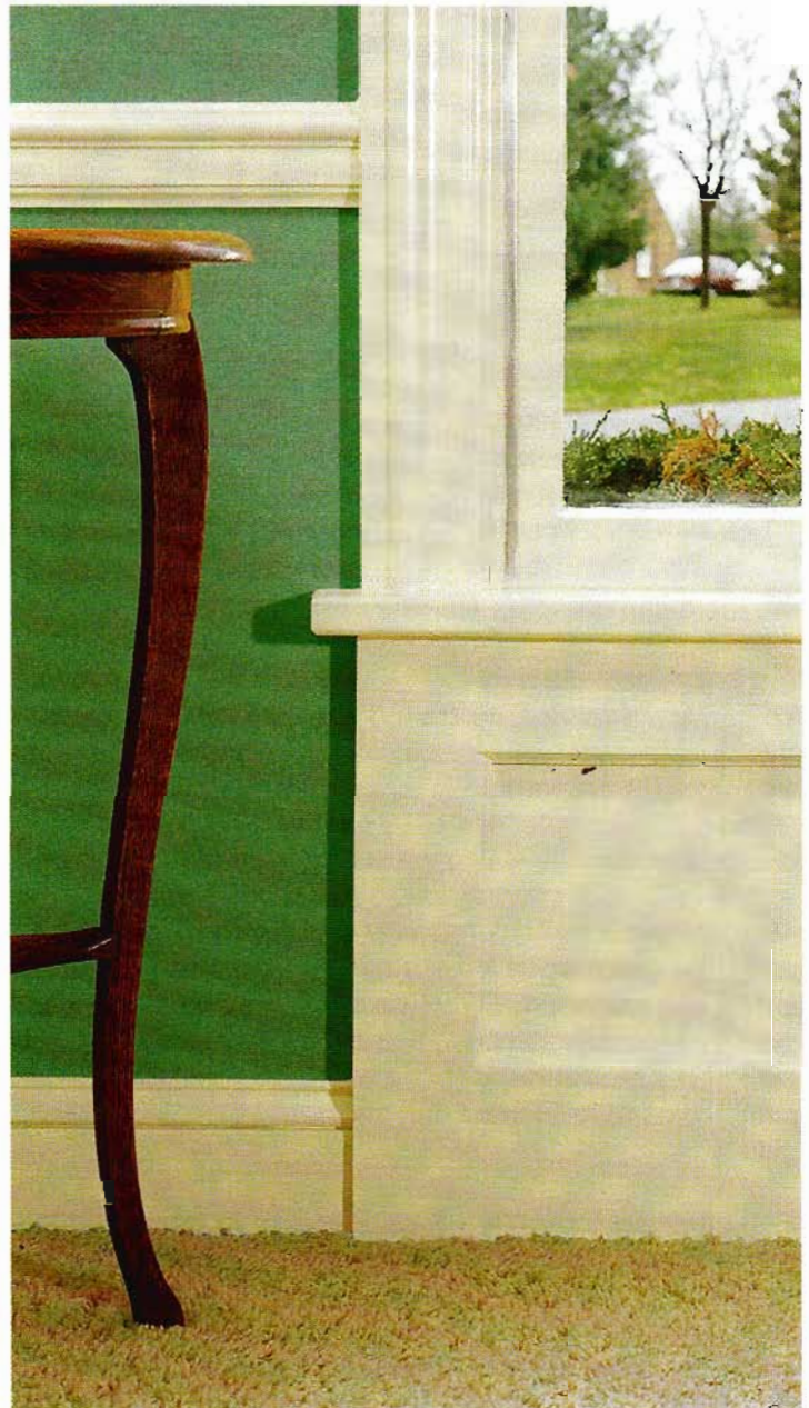
The horns of a window stool extend beyond the casing.
