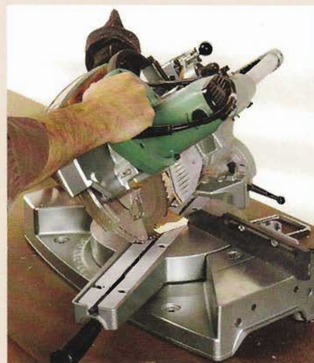
5 Cut an open miter to prepare for cutting the coped profile at an inside corner. Test the fit, and make necessary adjustments.
