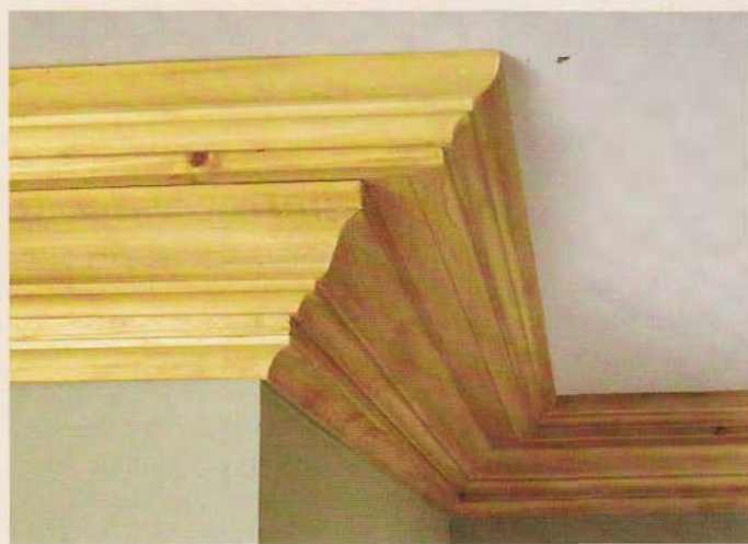
9 Completed built-up cornice. The goal is to make the multiple components look like one piece of molding.
