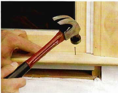
Finishing nails have a dimple on top to hold a nail set. When installing molding, the nail should penetrate into the underlying framing by at least 1 in.
