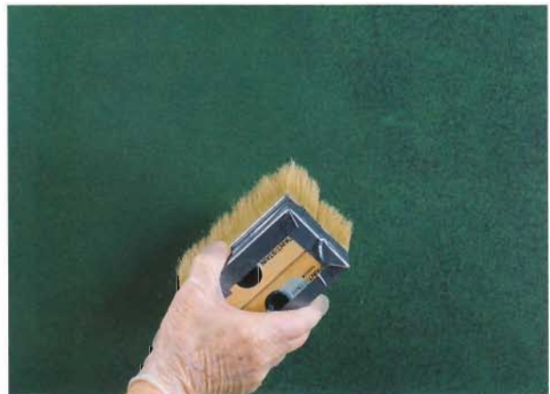
Stippling lends texture to a surface. Two taped-together staining brushes are an ideal tool.
