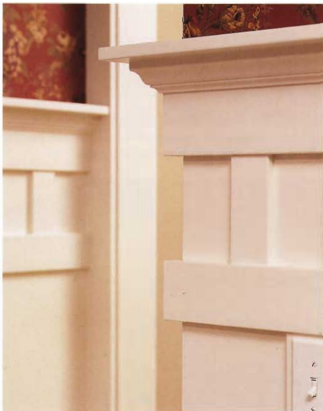
You can extend a basic chair rail with a plate rail, typically with a groove that holds plates propped up for display.
