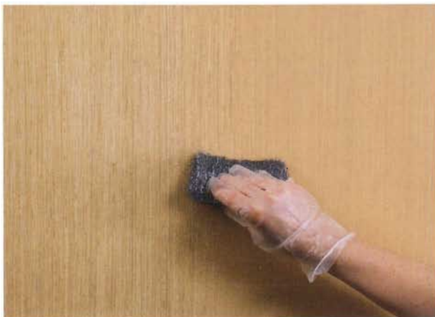
Combing techniques often imitate wood. Here a steel-wool pad is used to create the grain.
