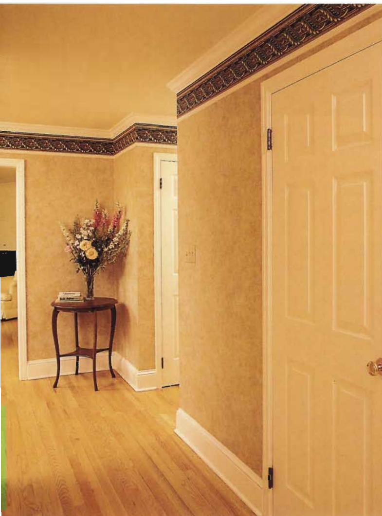
Long runs of molding , such as the crown molding along this ceiling, often consist of multiple pieces joined by scarf joints.
