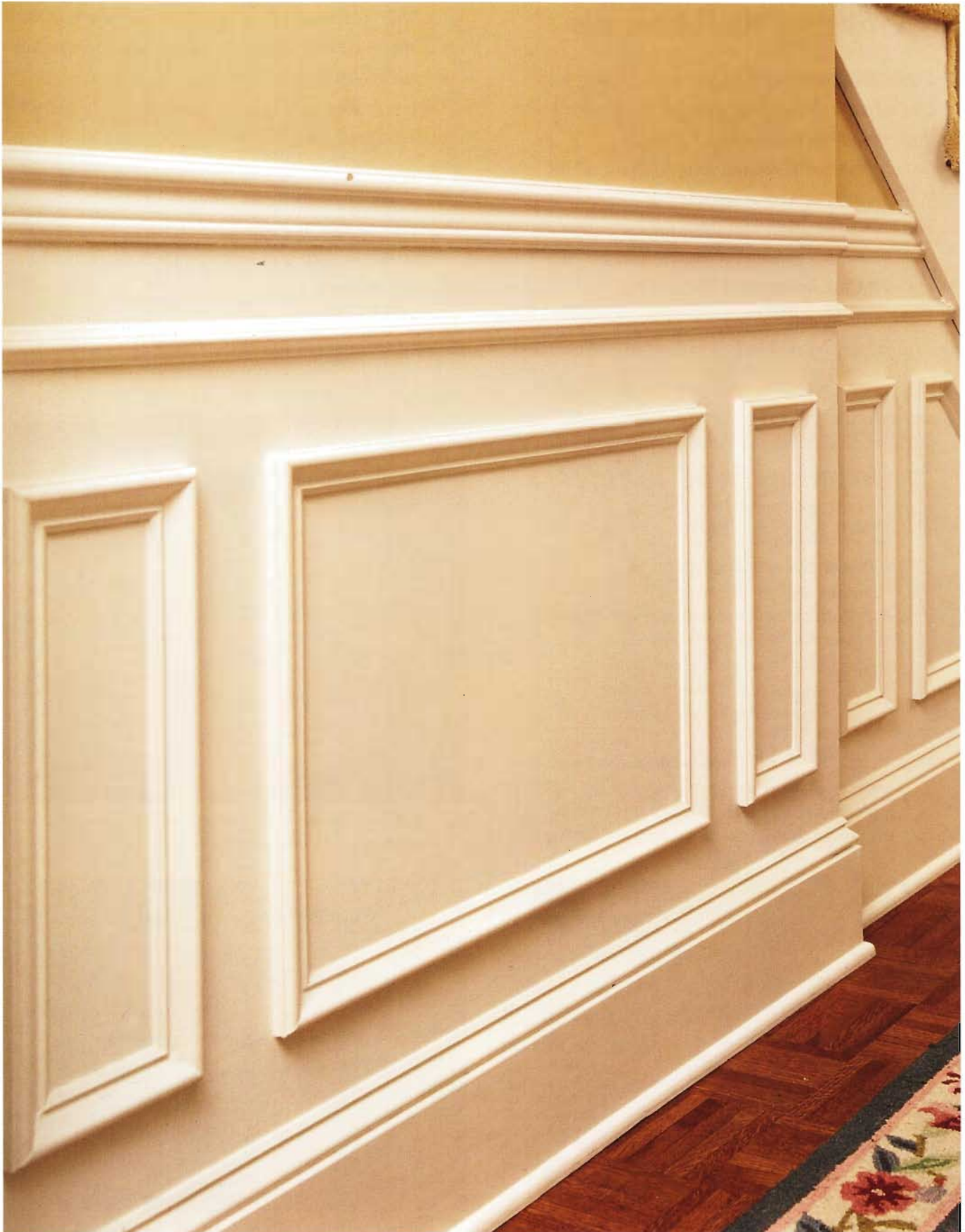
A single motif unit, which comprises a wide interval flanked by narrow intervals, is seen clearly on this wall.
