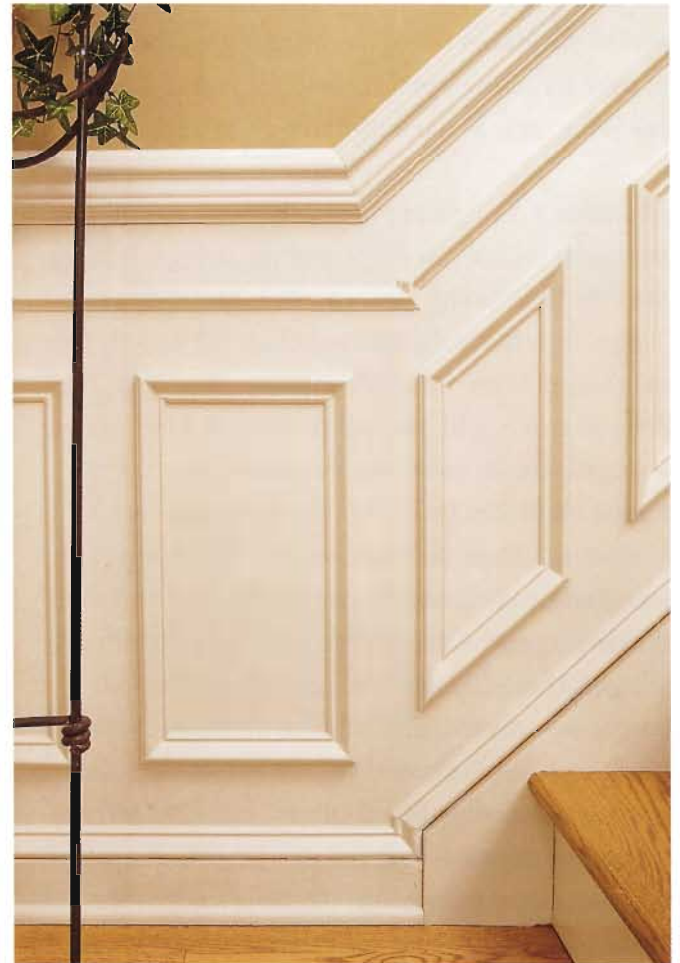
The smooth chair rail transition is possible because the stairway wall frames are smaller than those on the landing.
