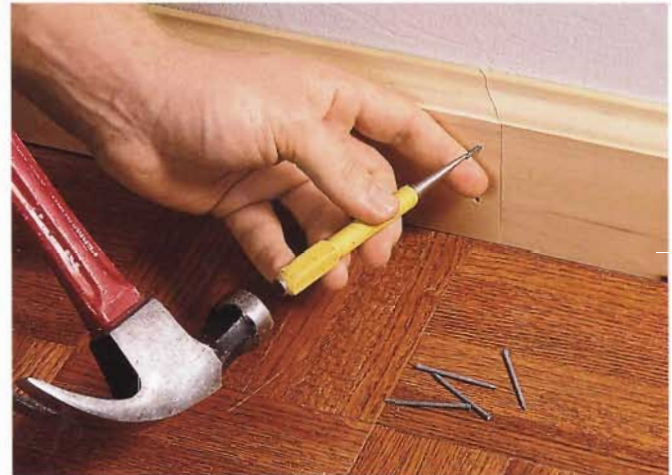
5 Drive finishing nails through the predrilled holes, and set the heads just below the wood surface.
