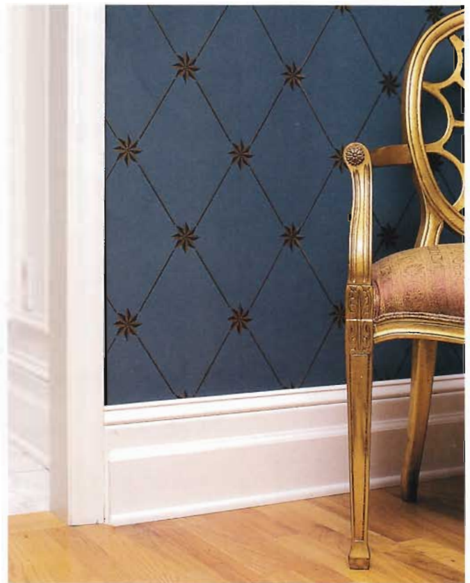
The built-up chair rail above combines a backer piece with narrower chair rail; a subrail runs beneath.
