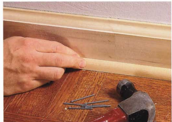
8 To further disguise the joint, consider nailing a shoe molding to the bottom of the baseboard.
