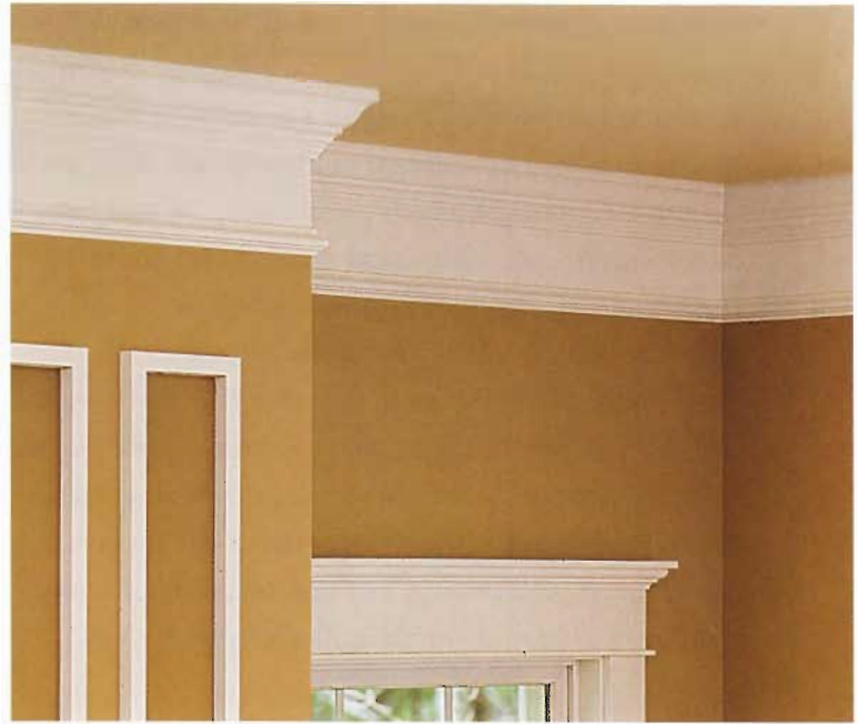
This large-scale cornice treatment consists of several stock moldings built up on a standard one-by-four board.
