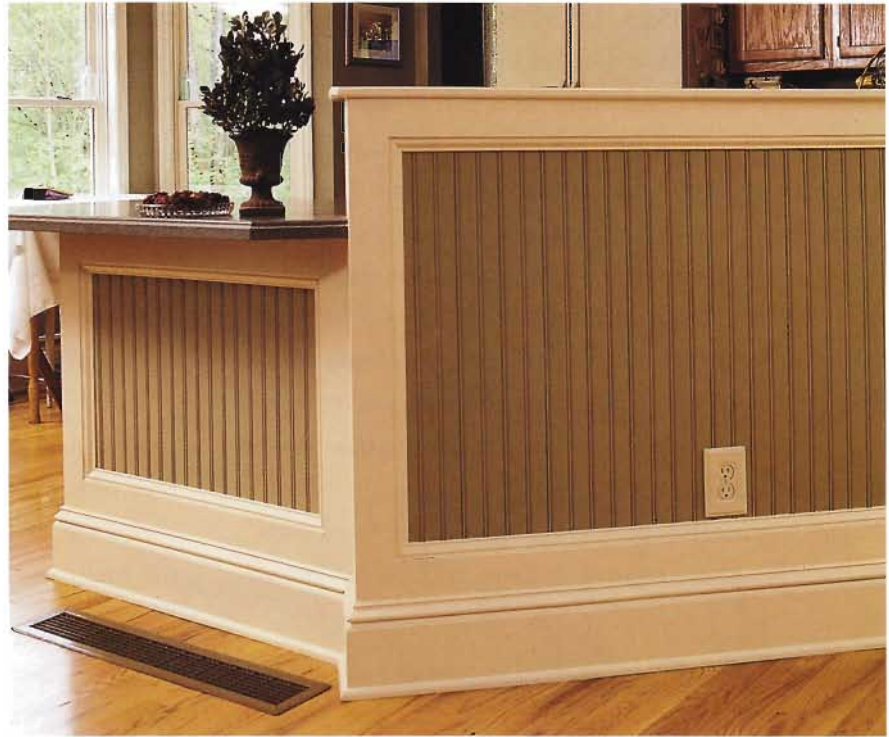
Finish base trim with shoe molding (often a quarter round) along the floor and base cap molding that matches the surrounding trim style.
