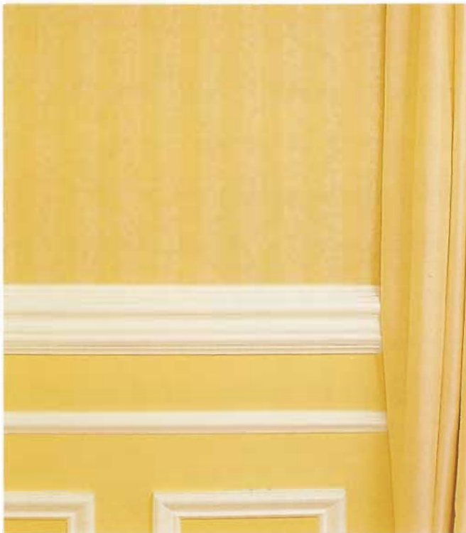
The built-up chair rail above combines a backer piece with narrower chair rail; a subrail runs beneath.
