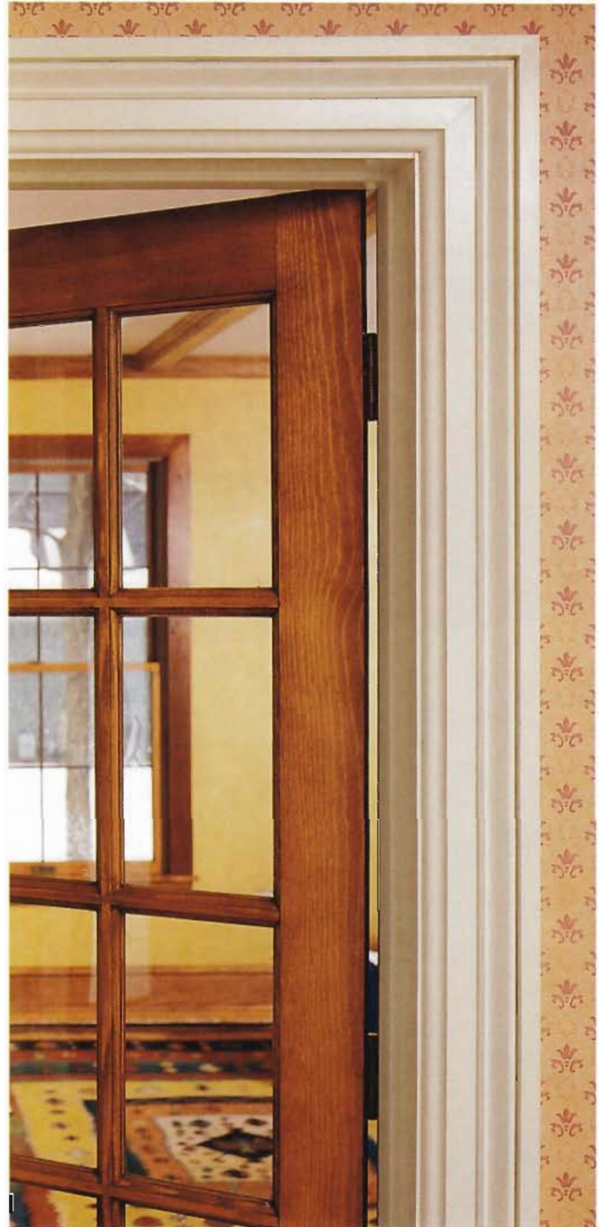
Built-up Colonial moldings add great depth and detail compared with smaller and plainer stock casings.
