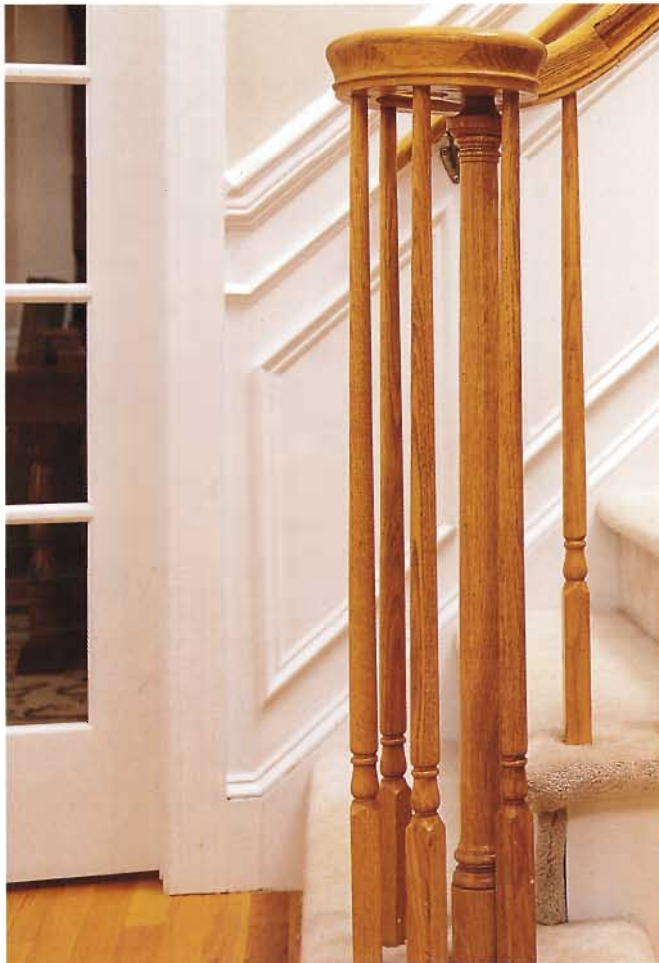
Door casings are sometimes a little too far for the chair rail to butt them; in these cases, the molding has to make a short jog.
