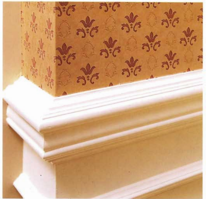
A chair rail makes a distinctive dividing line between flat-surfaced and framed sections of walls.
