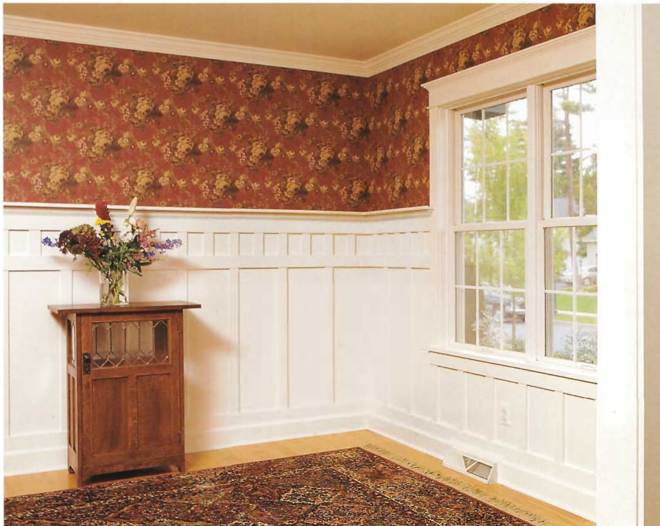
This wall treatment includes a subrail and upper midpoint vertical strips to create a decorative top section.
