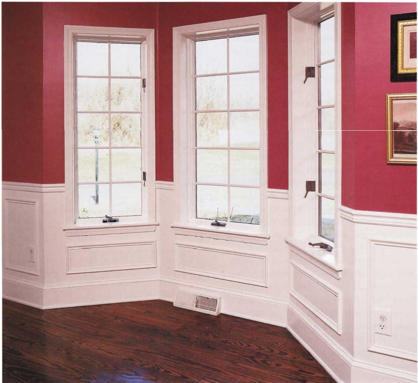
The wall frames in this bay line up with the window casings, and the vertical margins are wider than those in the rest of the room.
