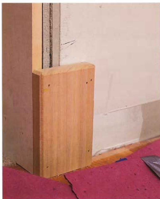
A plinth block at the edge of a passageway is chamfered on the side and top edges to provide a transition between the block and the fluted casing above it.
