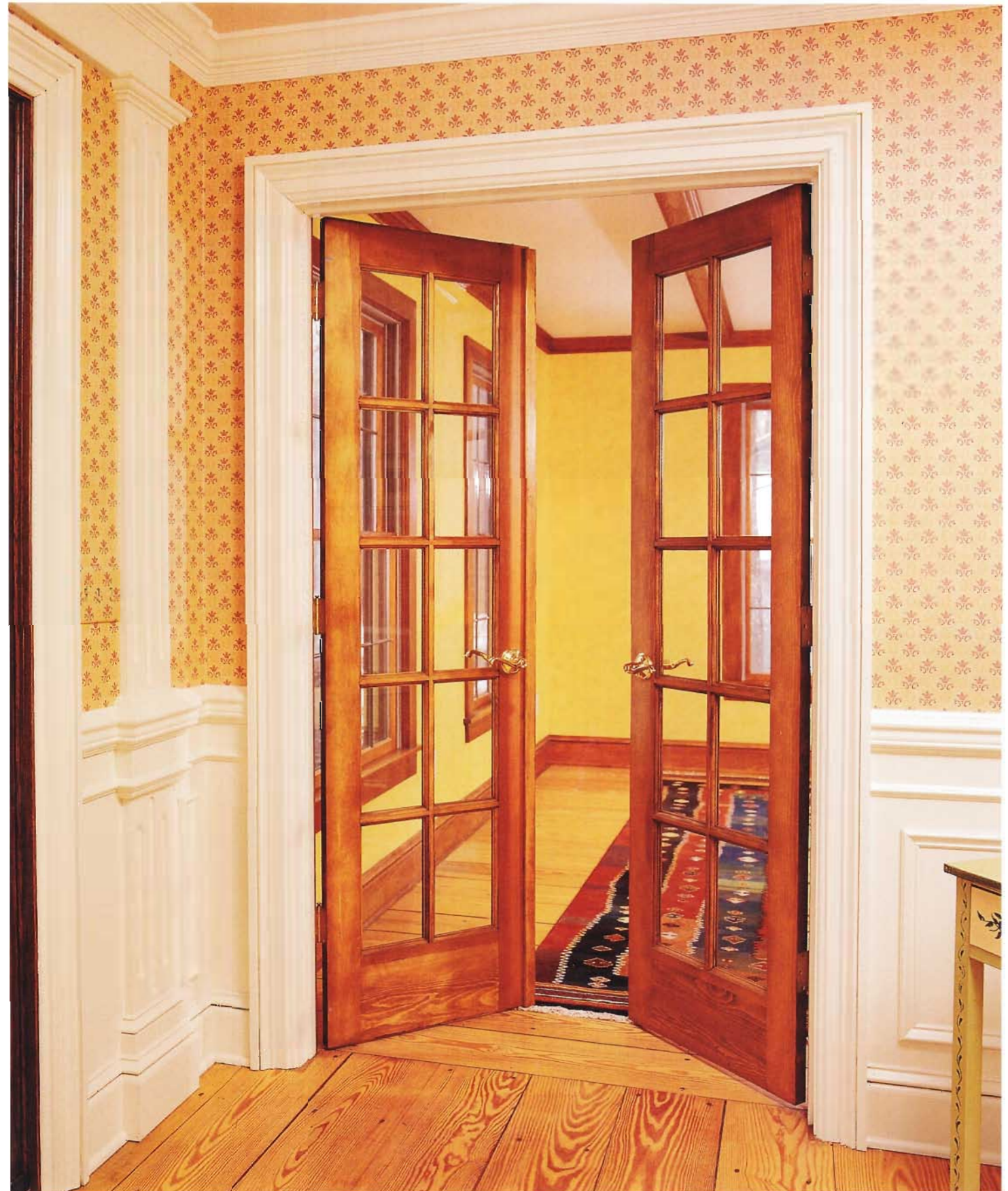
Door casings can be built up with molding, including an outer strip of backband molding, showing multiple reveals.
