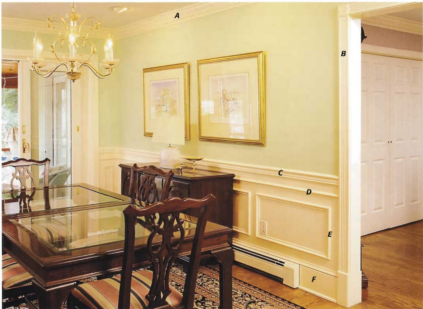
Different molding types include: (A) cornice; (B) door casing; (C) chair rail; (D) subrail; (E) wall frame; and (F) baseboard molding.
