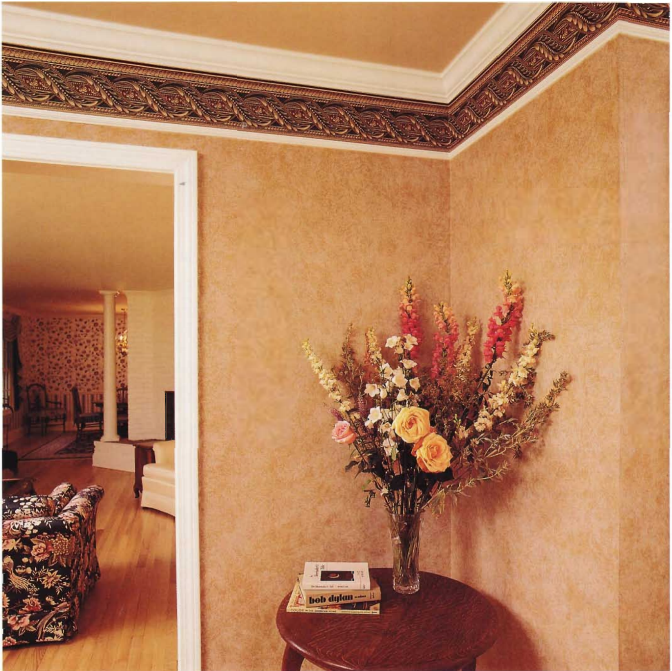
A layering of crown molding , a vinyl border, picture rail molding, and sponged-on wall color add drama to this room.
