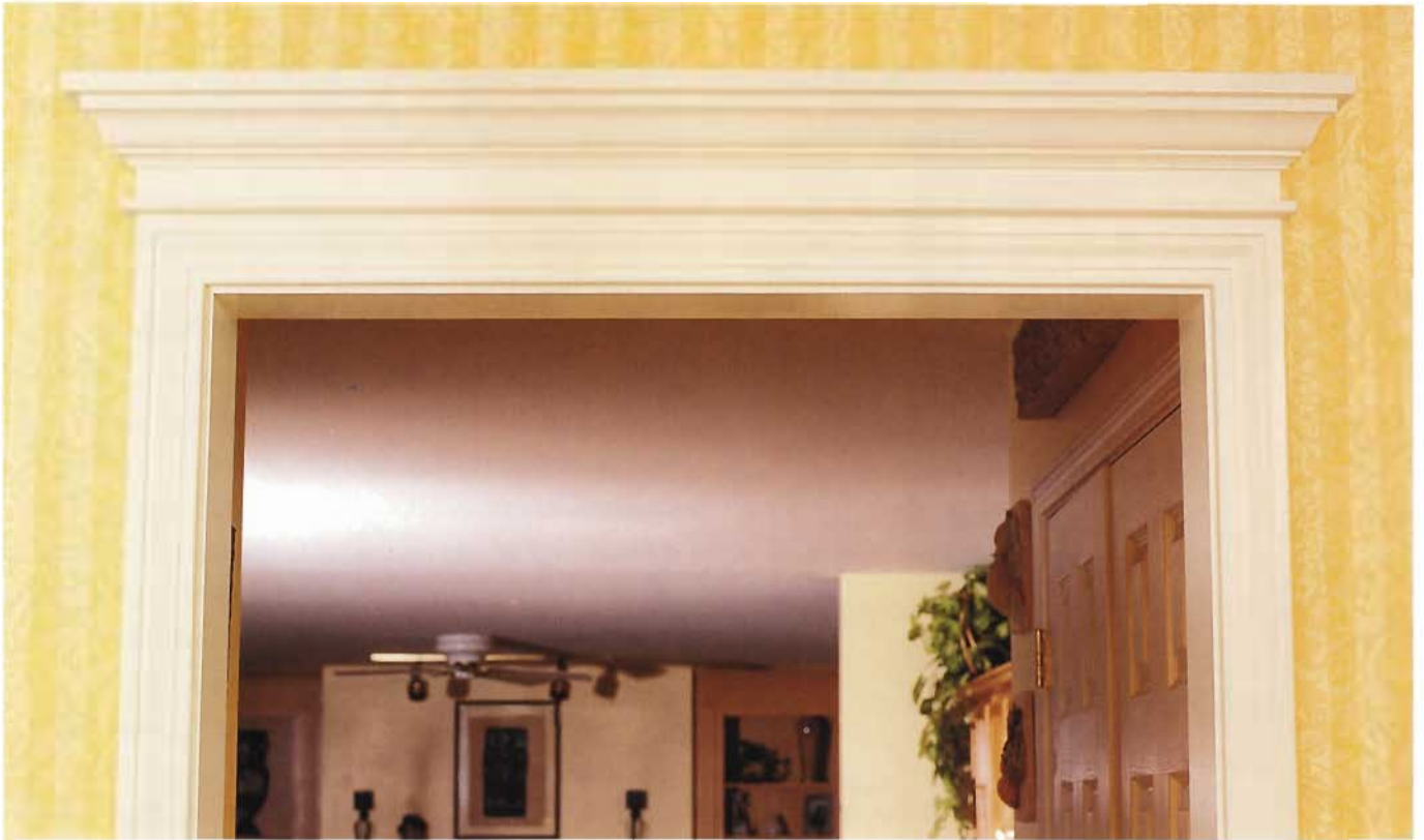
Decorative molding above openings can include a main crosshead trim piece, a frieze board, and a decorative cap.
