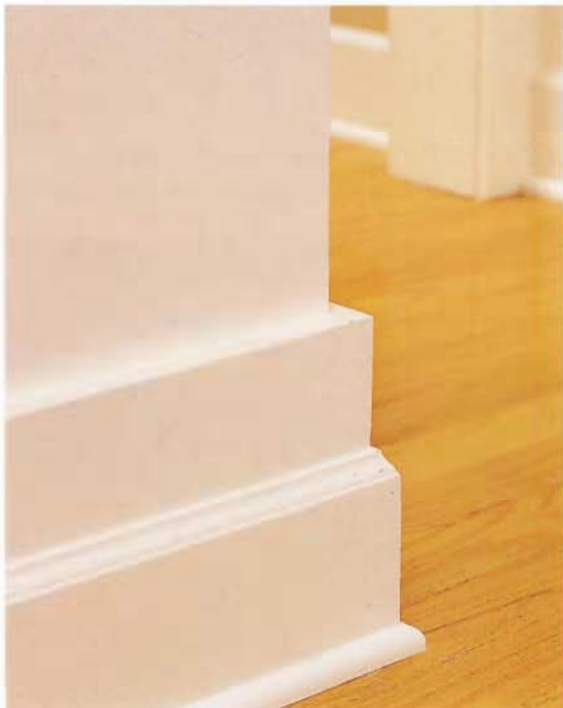
The base trim on this Arts and Crafts bottom rail is a simple baseboard with cap and shoe molding.
