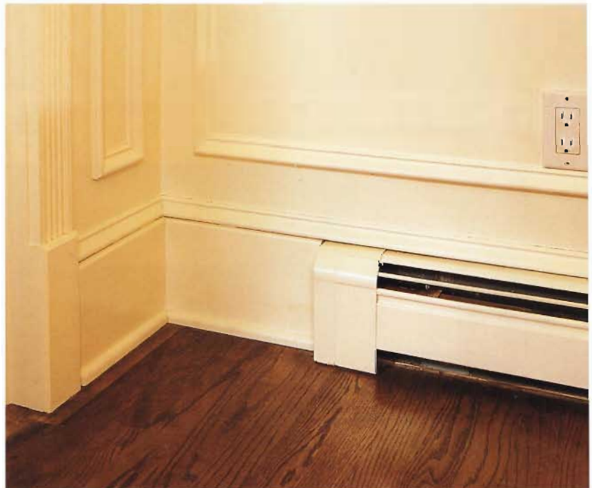
When you plan custom bases, consider the height of obstructions such as baseboard heaters or registers.
