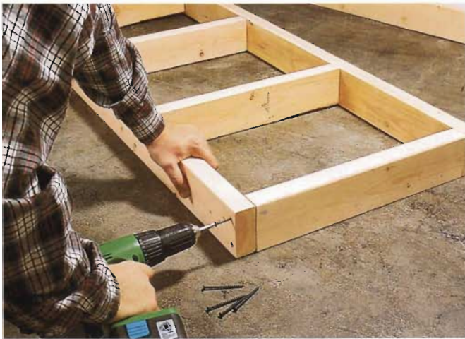
1 Make a strong and stable saw bench by framing the support platform with 2x4s on edge.
