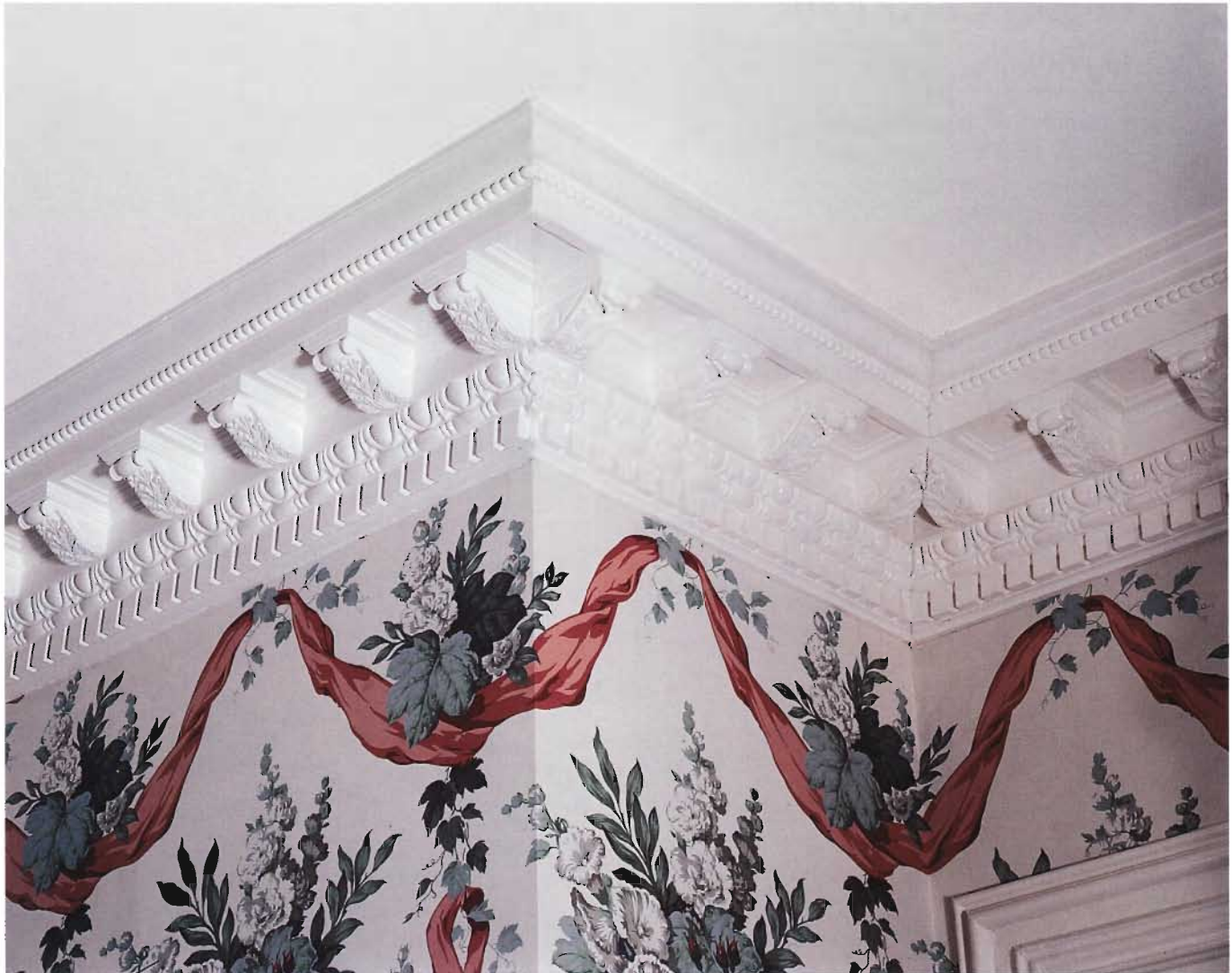
The intricate cornice above combines several moldings, including dentil block and egg-and-dart, for a formal look.
