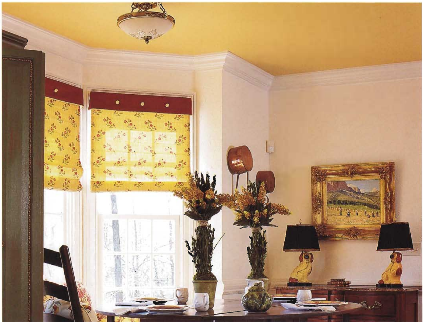
You need a variety of angled joints to continue crown molding around a bay window.
