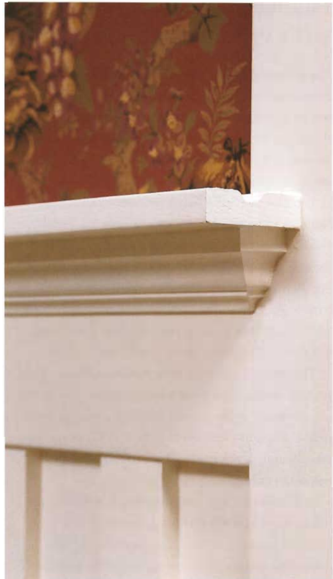
At plate rails that join door or window trim, ease the support molding onto the adjacent trim with a return.
