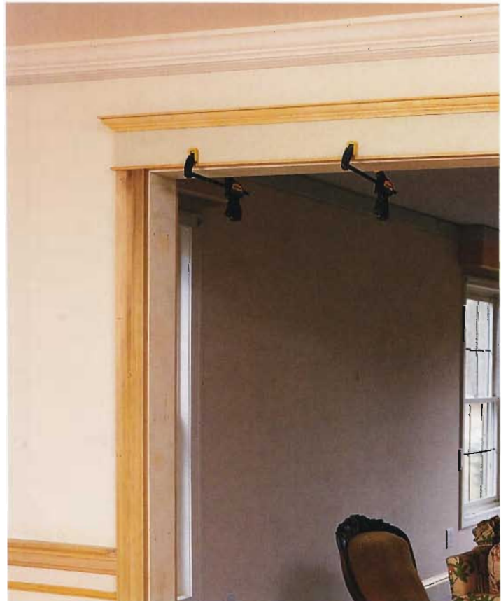
You can build the complete decorative crosshead assembly, above, on a bench. Clamp it in place on the jamb reveal line, right, as you fasten it to the studs.
