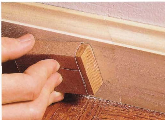
7 Clean up any traces of glue and filler around the joint with sandpaper before finishing the wood.
