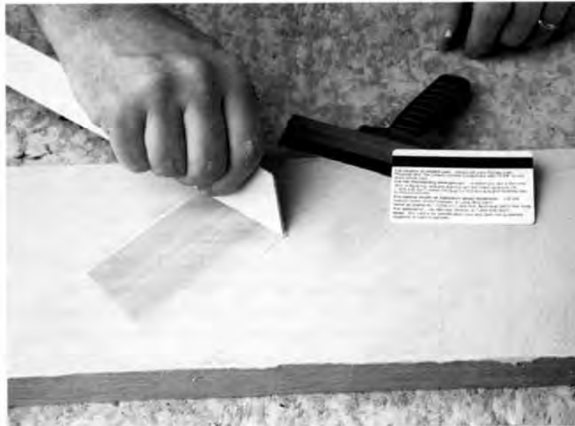
Rubber squeegees, plastic credit cards, and scraps of wood can all be used to scrape away excess filler. The point on the wood comes in handy when trying to dig filler out of deep corners.
