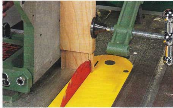
Remove the Edges. With the tenoning jig reset for the edge cuts, repeat the process for removing the waste, testing the fit as you go (photo at right).
