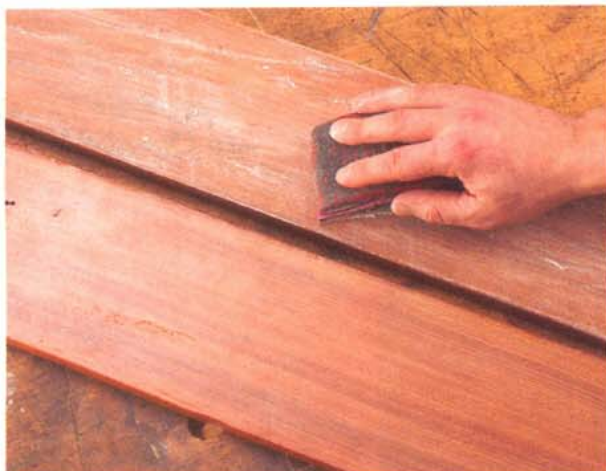
Sand out any unevenness and defects in the cured epoxy before applying the exterior varnish topcoats.
