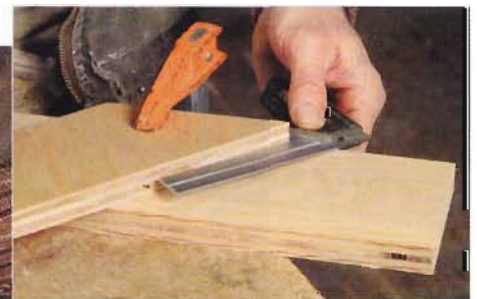
Clamp in place. Clamp components together to ensure that they are properly aligned (above). Keep components clamped as you drill holes and drive screws (left) to be sure the pieces don't shift.
