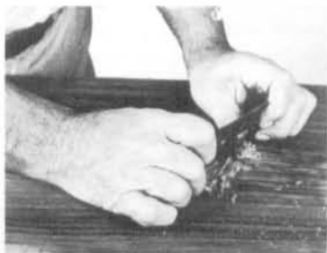
Block and clamp hold curly spot down while glue cools; strip of heavy paper along seam keeps it closed until glue dries. Then a sharp scraper cleans off paper and glue.
