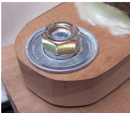
The pivot area has two ball bearings: one on top as shown and a second one on the bottom.
