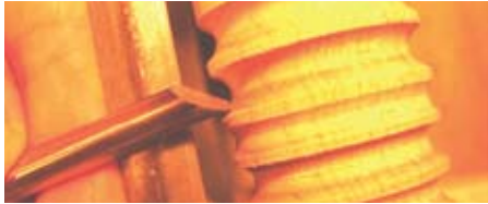
Fig. 2-4: Finishing the cove.
