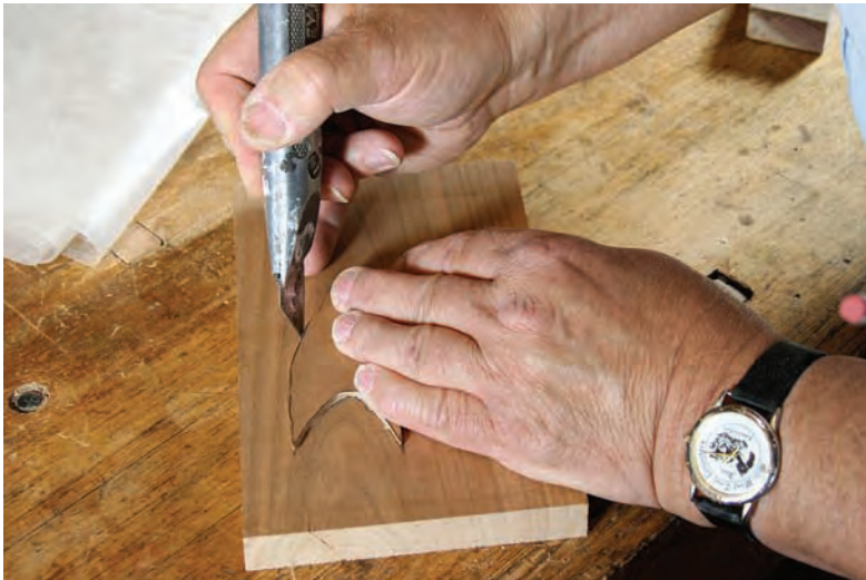
11 Tape and trace. Stick the patch down with cloth-backed double-stick tape. Trace around the undercut edge with a utility knife. Remember that you don't want the patch to be too thin. A thin patch will get torn up when you remove it.
