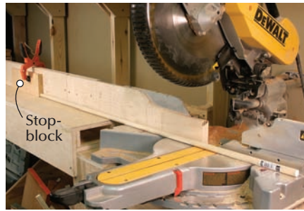
Stop-block. Here, I've set up a stop-block on the miter saw fence with a piece of offcut and a spring clamp. This saves a lot of time by not having to measure and mark each piece.
