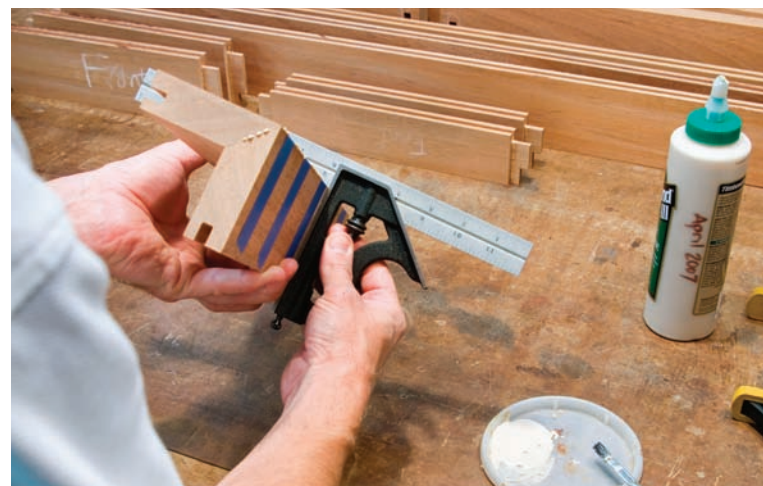
Mitered stiles. Both sides of the stiles at the corners are cut from a single, wide piece. The mitered edges are glued together with tape as a clamp.
