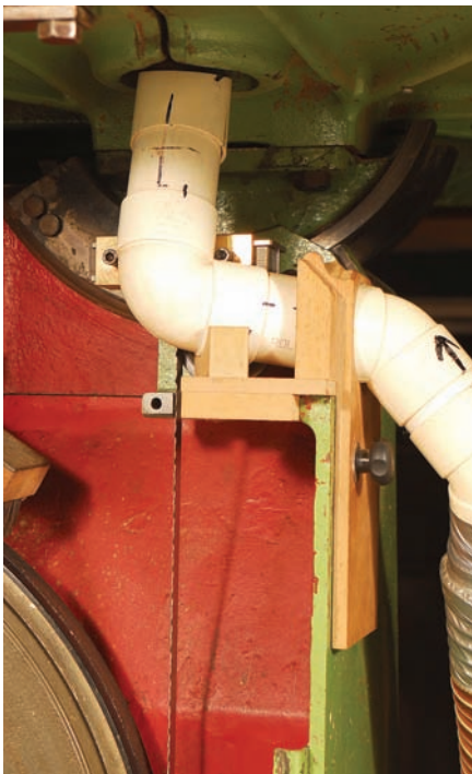
Custom dust collection. This “wrap around” dust extraction allows full table tilt to 45°. The door ledges stay clean!
