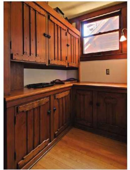
All in a row. The DeForest pantry cabinets featured stylized board-and-batten doors, and the numerous exposed screw heads are all aligned in the direction of the wood grain.
