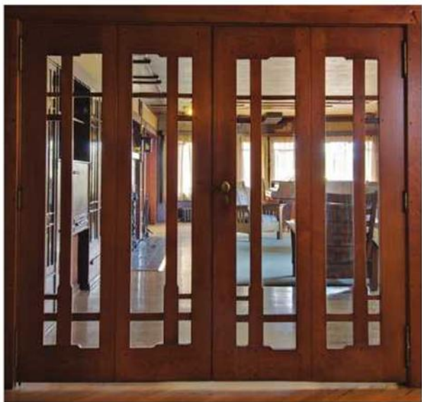
Unity, not division. The living room doors in the Thorsen house articulate spaces while continuing the overall design scheme.
