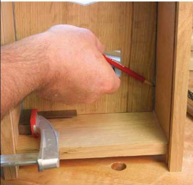
Where to position the supports. Hold the door closed and tight to a square, then mark the edges of the door. Use a folded business card to position the supports behind those lines.
