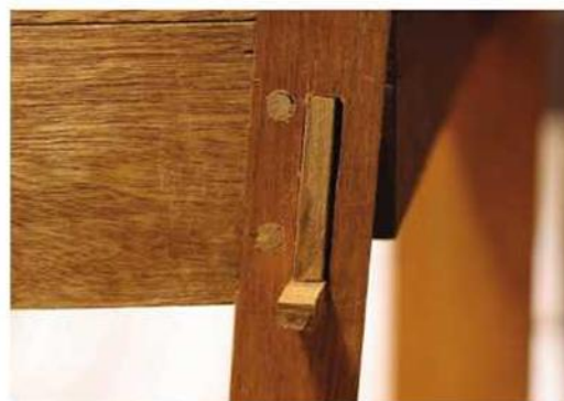
Tough job. This is the toughest joint in a chair full of tough joints. Something went terribly wrong marking out this tenon, but at least I got the rail positioned correctly! Turns out these tenons were typically wedged, but not with the massive \frac{1}{4} " block in this one. As bad as it looks now though, I'll bet it will look a lot better with a couple wedges and some leftover mahogany veneer from my standing desk. We may be surprised when it's done.
