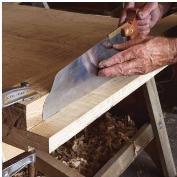
It starts with a saw. To make the breadboard end, I begin by sawing out the shoulder of the tenon. The block of wood acts as guide for the saw's blade.
