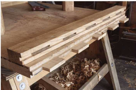
Ready for the pegs. In the finished breadboard end, you can see the stub tenon that fits into the groove and the five longer tenons.
