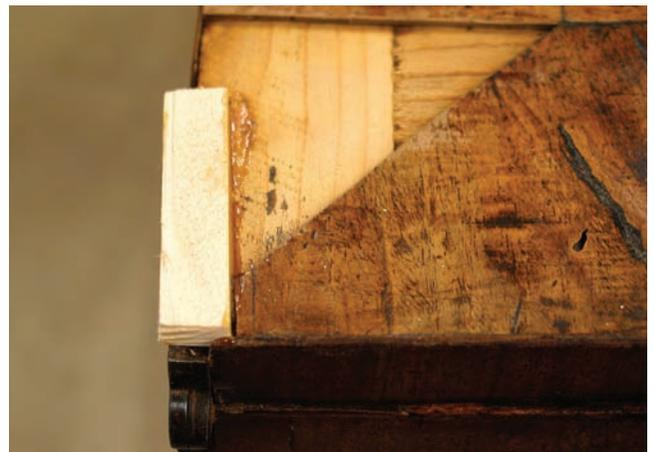
**6 Rub joint.** One of the reasons I love hot hide glue is that I can create a strong bond simply by rubbing two pieces of wood together with the glue in between. Work proceeds very rapidly using rub joints. Arranging a clamping setup for this patch would clearly be difficult.
