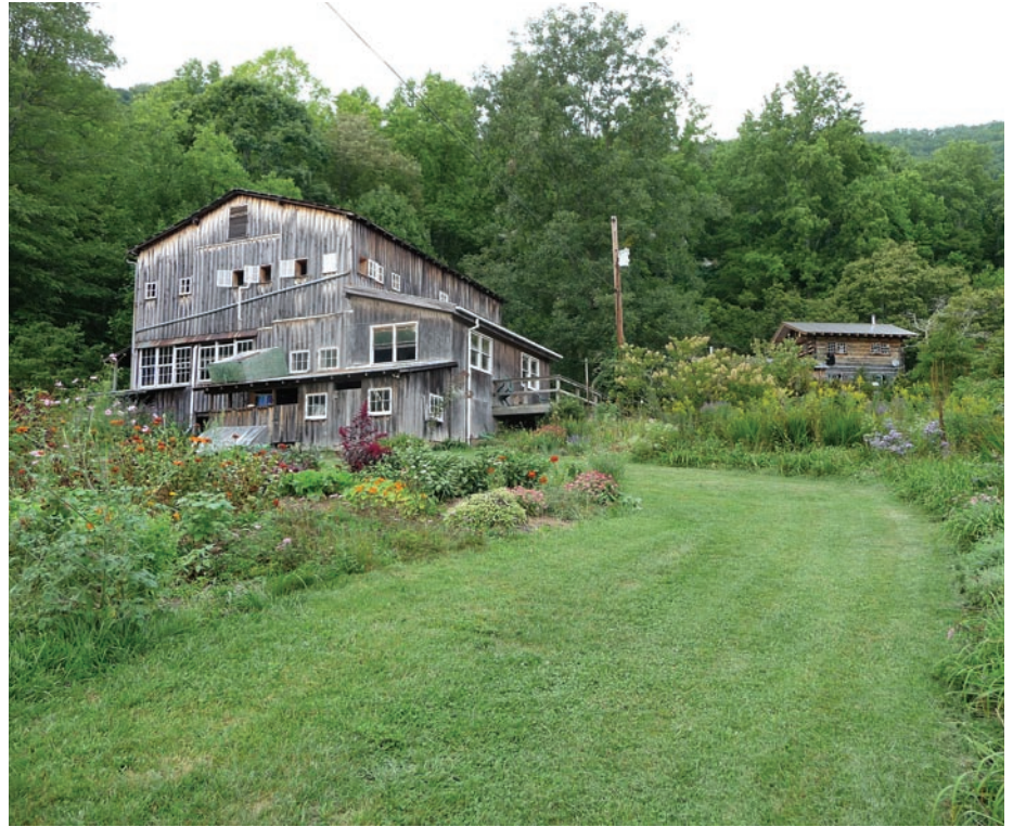
Country Workshops. Nestled in a beautiful Appalachian valley an hour's drive north of Asheville, N.C., Drew Langsner's school, Country Workshops, sits quietly in its stunning surroundings. The workshops and accommodations are in the converted tobacco barn (left), while Drew and Louise Langsner's home is farther up the hill (right).
