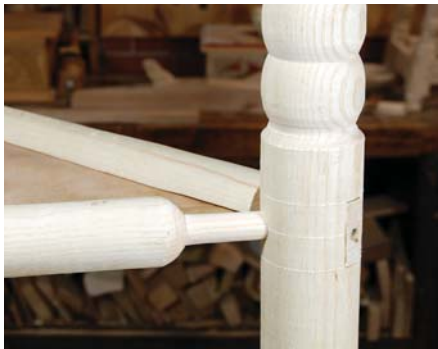
Tenons squared. Here, you can see the square tenon as it comes through the leg as well as the unseated round tenon on the adjacent seat rail. Each rail has one square and one round tenon.
