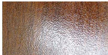
Orange peel. When the dots at the edge of a spray burst are large, you get an especially bad case of orange peel as shown here. Orange peel is so named because of the resemblance to the texture in the peel of an orange.
