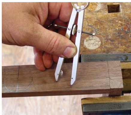
Cyma completion. Using a line scribed \frac{3}{4} " below the centerline, and the same compass setting, scribe the second part of the curve so that it blends with the first.
