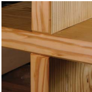
Make it a feature. Chamfering the edges add a design highlight – and helps to cover up any slight misalignment.
