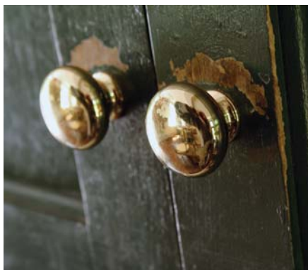
Open and shut case. Though fairly modern, these cabinet doors have been opened tens of thousands of times and show a typical wear pattern.
