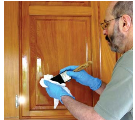
Brushing off excess. With the surface you want to cover wet with wiping varnish, begin removing the excess with single strokes using an almost-dry brush. Wipe the brush on a clean cloth after each stroke to remove the finish you just picked up with the brush.
