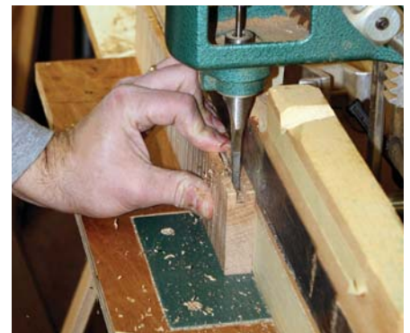
Joinery preparation. The mortises for the 1" door tenons are located at the bottom of the groove and completed with a mortiser.
