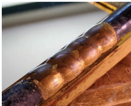
Overfed. This detail on a mirror has been coated with finish many times by an over-aggressive housekeeper.
