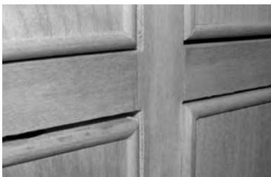
Cockbeading is a simple edge detail that can dress up doors, drawers and much more. But cutting this detail on a door panel can be a lot of work. The simple option is to run a quantity of 1/8"-thick hardwood through your router table adding a bullnose detail to one edge. Then, simply glue this edging to your panel. Presto – simple cockbeading.
