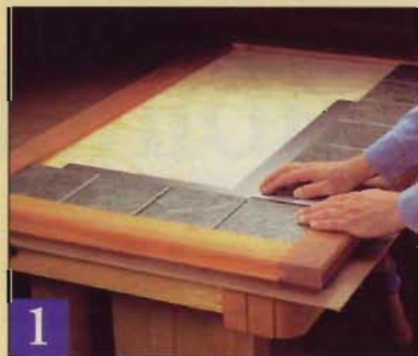
1 Set your tiles along two edges of the base. Use a framing square to keep the layout square as you space the tiles evenly.
