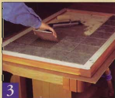
3 Place the tiles into the mortar with a small amount of pressure. Once the "L" is covered, continue working in small areas.
