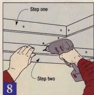
8 Screw the strips of drywall to the edges of the frames. Make sure the bottom edge of each strip is flush with the step.
