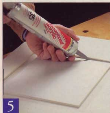
Applying caulk to the panel seams will prevent water from reaching vulnerable areas of your shutters and causing them to rot.
