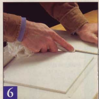
Improve the appearance of the caulk by wetting a rag and dragging it along each seam under the light pressure of your finger.
