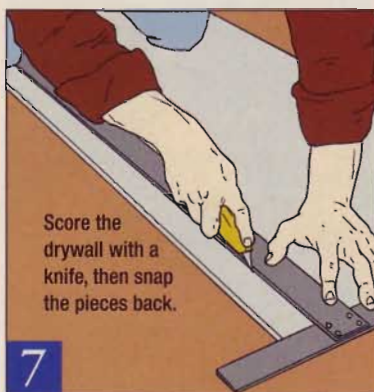
7 Cut narrow strips for covering the edges of each step. The traditional method calls for using a utility knife and a metal straightedge.
