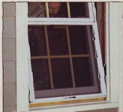
New windows in an old house, page 22.
