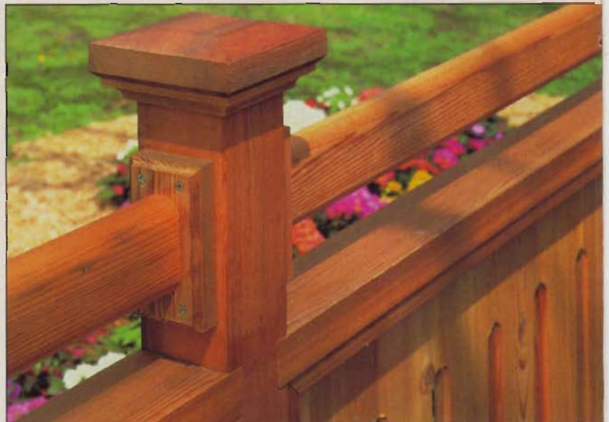
A new railing may build character into your old deck, page 16.
