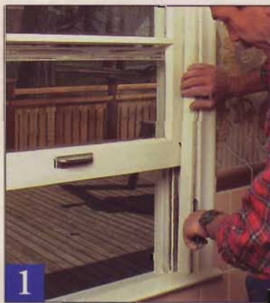
1 After scoring the paint or finish with a utility knife, use a small flat bar or putty knife to pry the stop molding from the window jamb.
