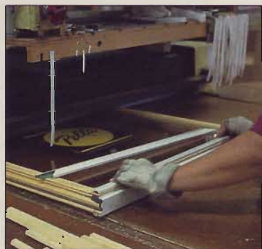
Mounting painted aluminum cladding to the exterior surfaces of the sash protects the wood during foul weather.
