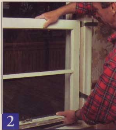
2 If your old window has a metal jamb liner instead of a parting stop, you may have to wedge the top sash free with putty knives.
