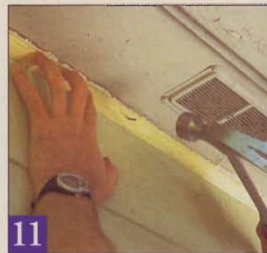
11 Because LockSide drops into place, you'll have a small gap above the top course. Nail molding in place to cover this space.
