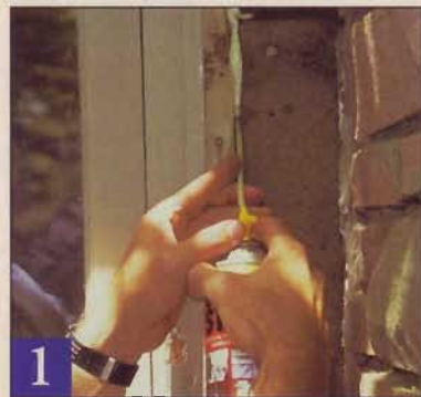
1 With the old siding removed, you may uncover gaps around windows and doors. Fill them with expanding foam insulation.
