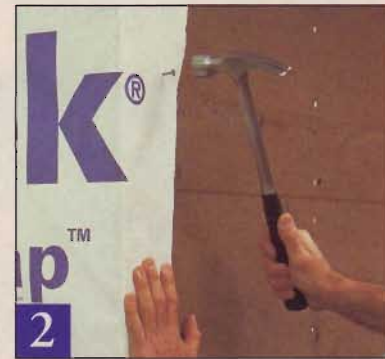
2 Housewrap installation should start at an outside corner, where the material can be overlapped. Fasten with nails or staples.
