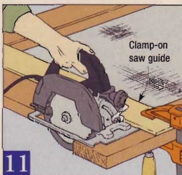
11 After checking your door opening for exact dimensions and angles, trim the door to fit. This removes the stile horns.
