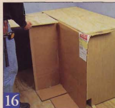
16 Use the cardboard cartons and some plywood to protect the base cabinets from damage while you install the wall units.
