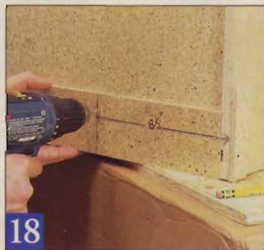
18 The cabinet and stud layout on the wall helps you locate the screw holes in each cabinet. Drill into the rails from the back.
