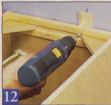
When you have the cabinets aligned and fastened together, anchor them to the wall. Place any shims over the studs.
