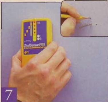
7 Use a magnetic or electronic stud finder to hunt for stud locations, then confirm each one with a nail test and mark the center.
