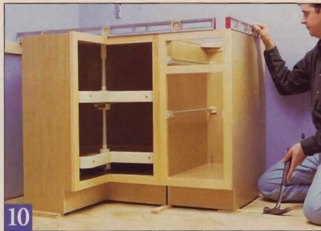
10 It may take some time to shim and adjust your first cabinets, but this step sets the precedent for everything that follows, so don't rush and expect to make it up later. At this stage, these units aren't fastened together.
