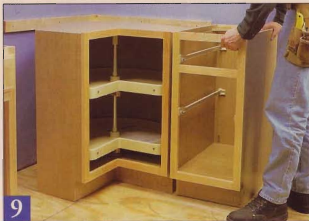
9 Do a test fit with the cabinets to identify any problems in the cabinet sizes or your layout marking. If its sides don't extend back to the wall, the corner cabinet will have to rely on adjacent units for correct positioning.
