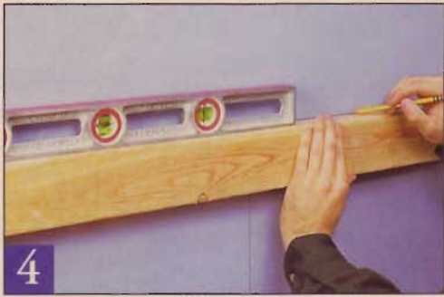
4 Using a long level and a straightedge, mark a continuous line from your 34½" reference point. This is the base cabinet level line. Mark another line 19½" higher.
