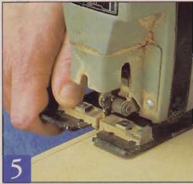
Use a jig saw to cut the substrate roughly to your scribe line, keeping to the waste side of the scribe line.
