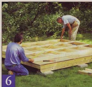
6 Secure the girts with a single nail at each end, then measure the frame diagonals. When you're squared up, nail in the girts.
