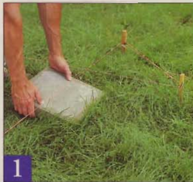
Position the concrete pads so they'll be centered directly under the skids. All nine pads must be level with each other.
