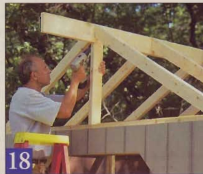
18 After you install the common rafters, add the ridge posts, gable struts, and the upper siding.
