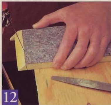
Miter the end of the backsplash, then use a coping saw to trim away the excess, following the edge of the laminate.
