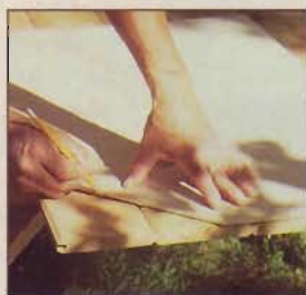
Scribe a template from the top of the door frame, then use it to lay out and cut the doors.
