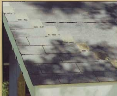
Offset the end joints of each course 6" from the one below. You can use the remnants from cut shingles as starter pieces above.
