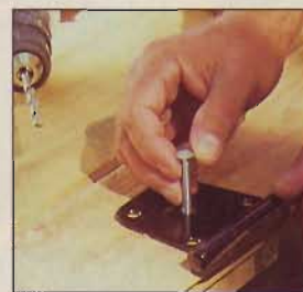
For added security, we substituted a 1/4" carriage bolt for one of the hinge-plate screws.
