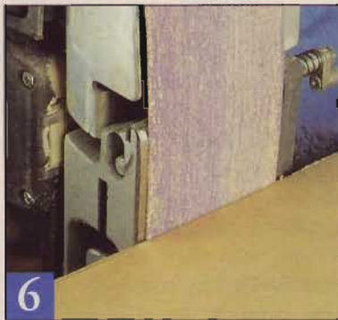
Complete the trimming to the scribe line using a belt sander. Tilt the sander slightly to undercut the edge for a better fit.
