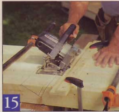
15 Clamp the rafters together to gang-cut the 30° plumb cut for the bird's-mouth. Use a jig saw for the seat cuts, one at a time.
