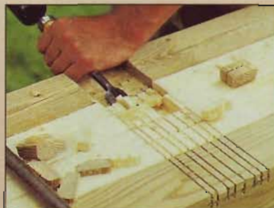
With the scoring cuts done, the bulk of the waste will break loose. Use a chisel (bevel up) to do most of the clearing work.
