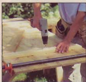
Screw horizontal and diagonal braces to each tongue-and-groove cedar door panel.
