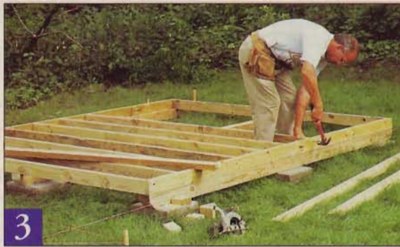
After you mark the layout lines on the two rim joists (indicating the location of each floor joist), nail the platform frame together.
