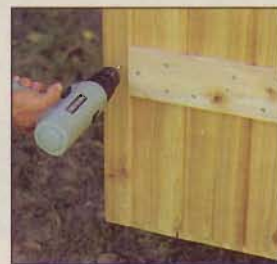
A narrow wood strip, called an astragal, bridges the door gap. Fasten it to the left-hand door.
