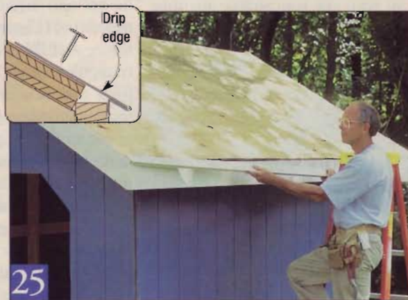
25 Aluminum drip edge flashing will keep water runoff away from the wood fascia. Nail it to the sheathing before the felt goes on.
