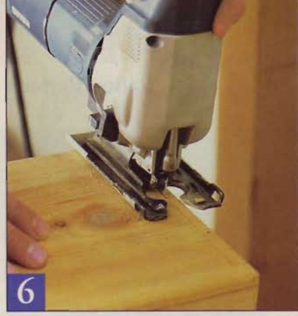
6 Cut the ends of the beams to the siding profile using a jig saw. Apply outdoor oil finish to the freshly cut end grain.
