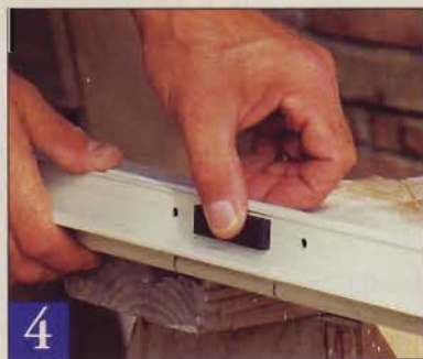
4 To adjust the fit and add support, install shims on the back of the hinge jamb between the mounting screw holes.
