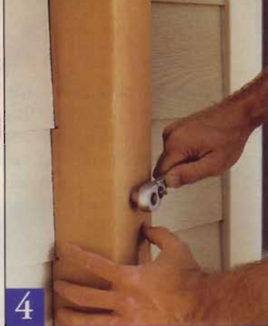
4 Drill counterbored holes in the post, followed by through-holes in the post and siding. Next, install the toggle bolts.
