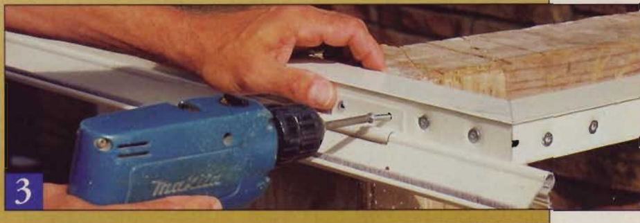
1 Cut the hinge jamb to length, angling the cut on the bottom end to match the slope of the door sill. Support the aluminum frame with a wood block. 2 Position the hinge jamb on the door to create a \frac{3}{16} " head gap, then 3 drill holes and drive the hinge screws.
