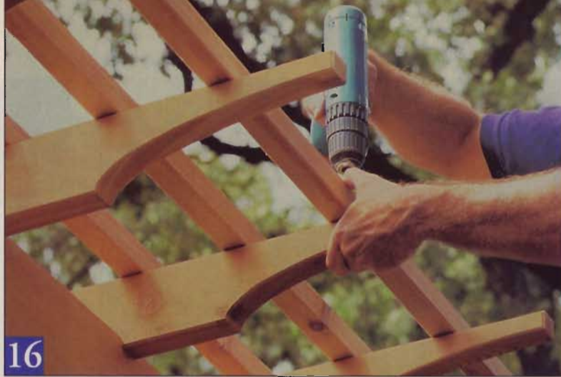
Attach the slats to the rafters with 3" deck screws. Position the slats so end-to-end joints are butted tightly together and fall directly on top of the rafters.
