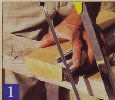
1 Cut the hinge jamb to length, angling the cut on the bottom end to match the slope of the door sill. Support the aluminum frame with a wood block. 2 Position the hinge jamb on the door to create a \frac{3}{16} " head gap, then 3 drill holes and drive the hinge screws.
