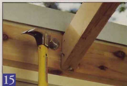
15 Toenail the rafters to the ledger, nailing them from the bottom first — this holds the rafter in proper alignment. Then toenail through the rafter from both sides, offsetting the nails.
