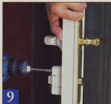
9 With the mounting holes drilled, install the latch and deadbolt assemblies. Snug up the screws to hold them in place.
