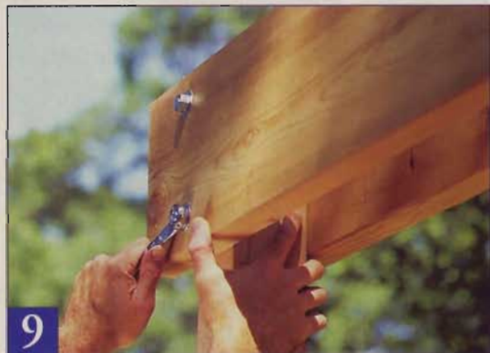
9 With the beams hoisted into position, tighten the carriage bolts that hold the beam assembly to the post.
