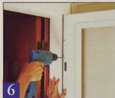
6 Open the door and drive mounting screws into the side of the hinge jamb. Don't overtighten them — you could bend the jamb.
