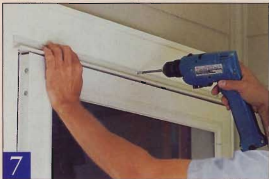
7 Position the head jamb above the hinge jamb, establish a uniform \frac{3}{16} " gap, then mark the mounting hole locations. Drill pilot holes and drive the mounting screws.
