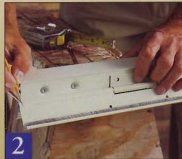
1 Cut the hinge jamb to length, angling the cut on the bottom end to match the slope of the door sill. Support the aluminum frame with a wood block. 2 Position the hinge jamb on the door to create a \frac{3}{16} " head gap, then 3 drill holes and drive the hinge screws.
