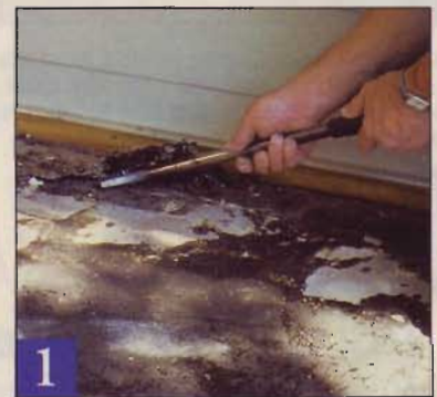
1 Scrape off loose materials then scrub the concrete with soapy water and a brush, leaving a clean surface for the mortar.
