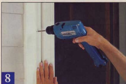
8 Set the latch jamb in place, establish a uniform \frac{3}{16} " gap, and mark the screw hole locations. Drill pilot holes and install the screws, checking the gap as you work your way down.
