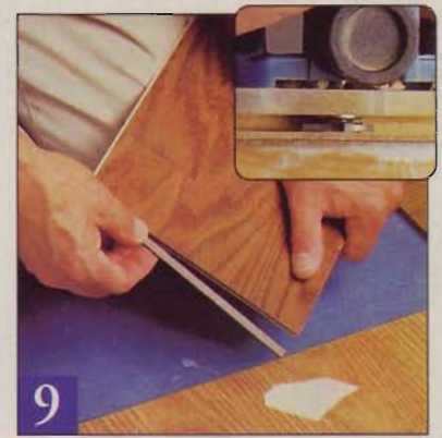
9 Use the bit supplied by the manufacturer to cut a groove in the trimmed piece. Glue the spline in place, then install the plank.
