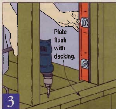
3 Drive screws through the back wall sill plate into the deck joists. Check the wall for plumb with a level.
