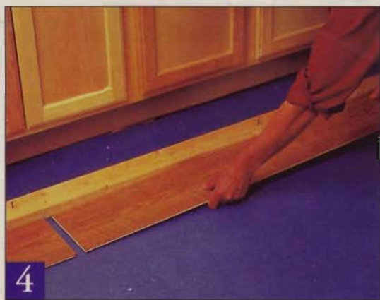
4 Lay the grooved edge of the first row of planks against a cleat tacked along the baseline. Remove the cleat and fill in the outside edge once the rest of the floor is down.
