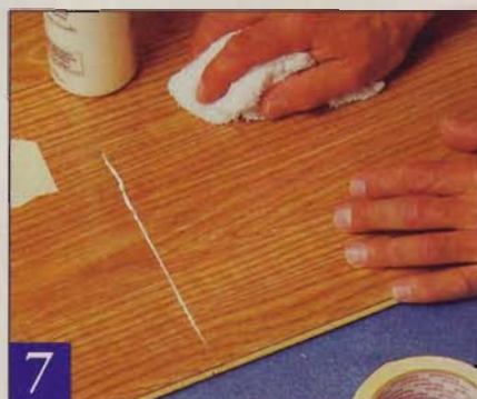
7 Wipe up any glue squeezeout with a damp rag, and rinse it often to avoid leaving a film. Masking tape holds the joints while the glue dries.
