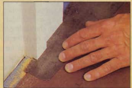
To trim door casing, lay a piece of flooring, laminate side down, on top of a piece of backing pad. Then use a hand saw to cut the casing.
