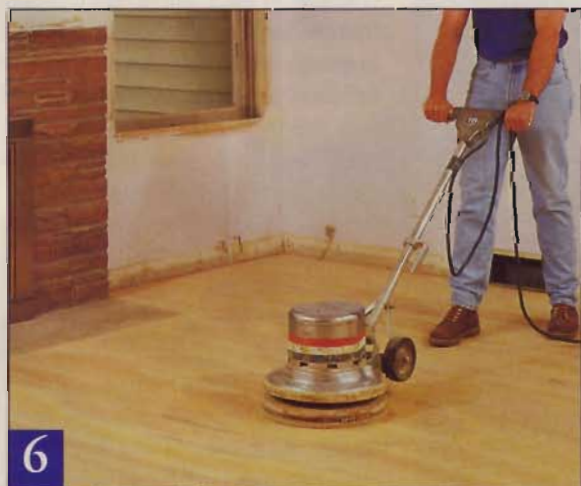
6 A floor polishing machine, fitted with a fine-grit abrasive screen, does a nice job cleaning up heavy scratches from the belt sander.
