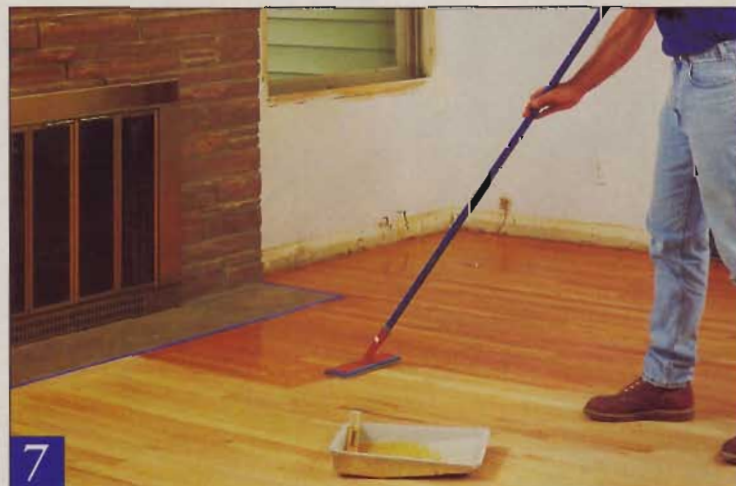
7 A paint pad or lamb's wool applicator works best for applying the finish. Never use a paint roller for this — it agitates the finish and creates air bubbles.
