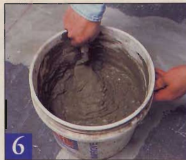
6 Mix dry latex-modified mortar with water, then let it stand for 10-15 minutes.
