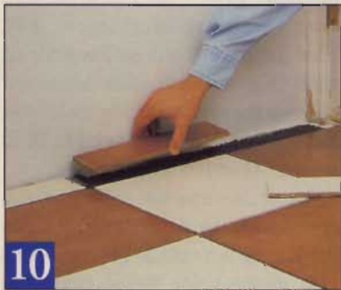
10 Even the best layouts may require narrow tiles. Hide them in inconspicuous places.
