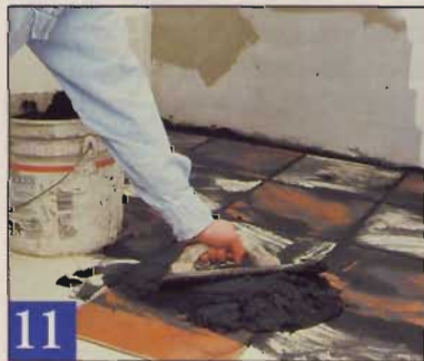
11 Spread grout with a float — diagonal passes avoid lifting grout out of joints.
