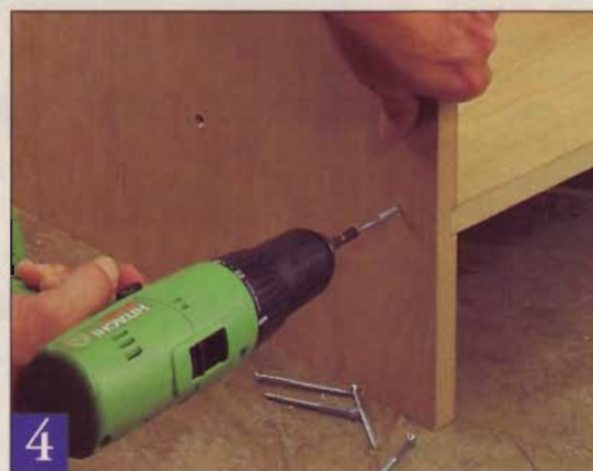
4 After spreading glue in the dadoes, put the panels together and drive screws into all the joints. The screws will draw the panels tight together without the need for clamps.
