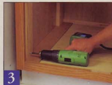
3 Using #8 x 1" flat-head screws, fasten spacers to the cabinet. To avoid splitting, first drill countersunk pilot holes.
