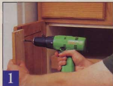
1 After removing the stile, screw it to the back of one cabinet door. It will fill the gap between the doors when they're closed.
