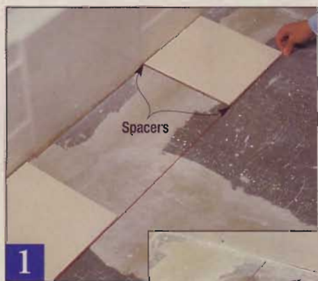
◀ To create a baseline start by setting two tiles against a straight feature in the room (the bathtub, in my case). Placing spacers on either side of the tiles allows for grout joints, then you can snap a chalk line.
