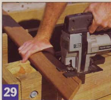
The first piece of ribbon decking, like others around the edge of the deck, gets notched to fit around a post.
