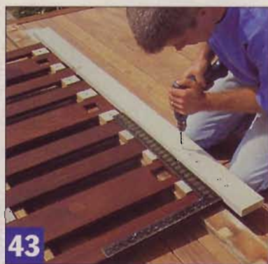
43 Uniform spacing between balusters is achieved with a simple jig. Check the assembly for square before fastening.
