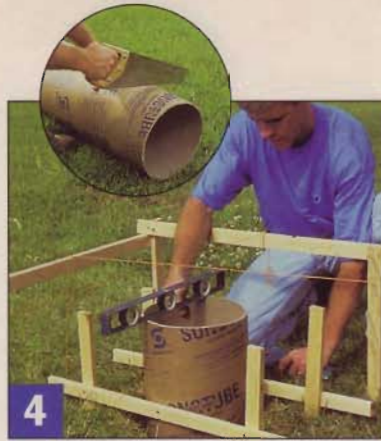
4 Use stakes and crossbars to suspend the footing forms about a foot off the bottom of the hole. Drive 1 1/4" screws to hold the form level in one direction.
