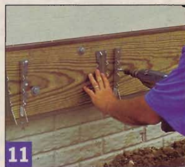
11 Metal hanger brackets will support the deck joists at the ledger. Nails don't hold as well and tend to squeak after a while, so use screws to fasten these.
