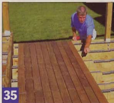
Once the decking section outgrows the clamp reach, skip one course and snap a line to start another section.
