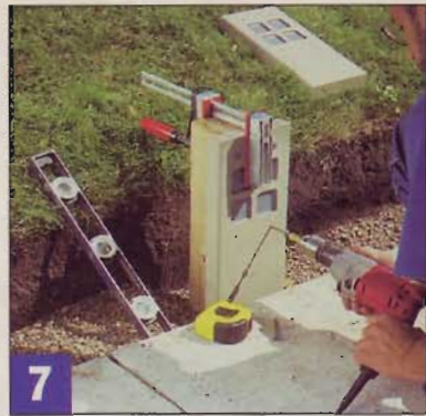
7 The fascias bear the wall's load directly, so use serious fasteners to secure them to the posts. I got RSS structural screws from GRK, (800) 263-0463.
