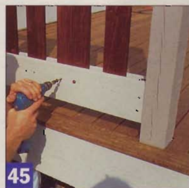
45 Add the cedar rails on the outside to close up each railing section. Painted GRK screws add to the design.
