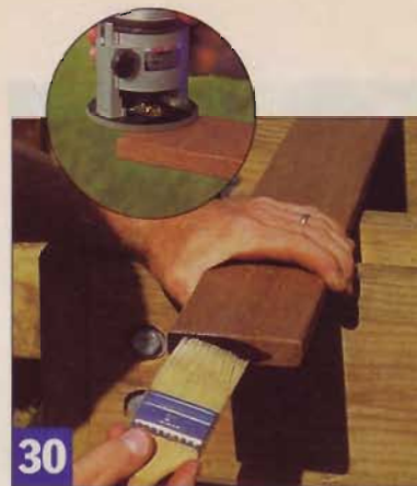
After routing all the cut edges of the decking with a small roundover bit, apply sealer to the end grain.
