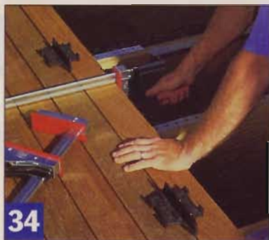
Clamps can coax crooked boards into a straight line before you fasten them. Always use spacers for a uniform gap.
