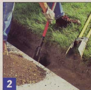
As you dig each post hole, shape the sidewalls like a wedge, wider at the bottom and tapering toward the top.
