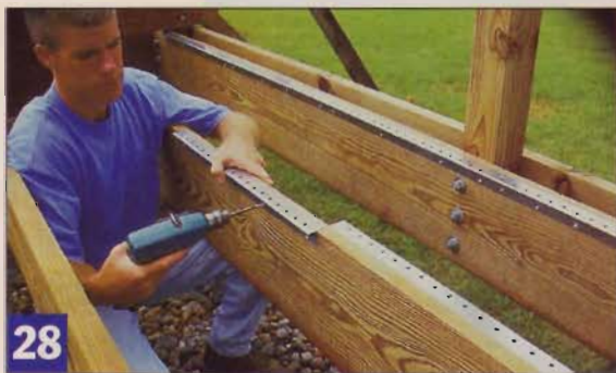
DeckMaster brackets get fastened to the joists from the side. Use the holes on top to secure the decking.
