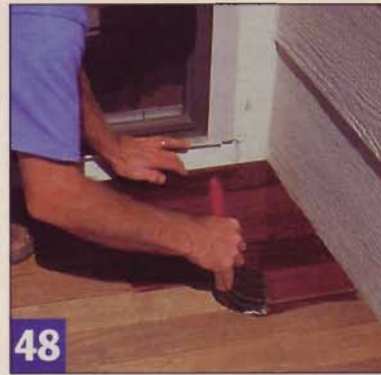
48 For a final touch I applied Penofin oil finish. It brings out the ipe's rich color and will help protect the wood.
