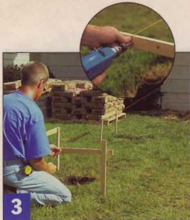
3 Tie strings close to their final location and check for square corners (see Skill-BUILDER). Drive screws to mark the centers and edges of the posts.
