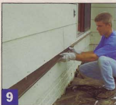
9 Whether or not you remove the siding behind the ledger, tuck metal flashing under the siding course above it to divert water away from that area.
