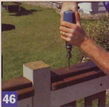
46 After fastening the 2x6 rail cap to the cedar rails, add the 1x4 rail trim. Routed edges offer a friendlier touch.
