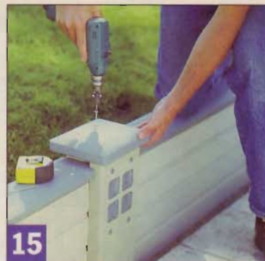
15 The post caps install the same way. You should have about a 1" space between them and the rail caps below.
