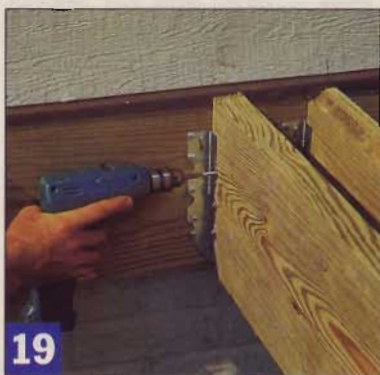
19 Use screws to secure the joists in their hanger brackets, and fasten at each hole for maximum holding power.
