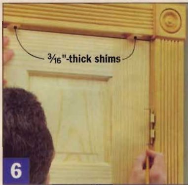
6 Hinge alignment demands precise marking and cutting. Avoid measuring errors by shimming the door in place and marking each hinge location directly.
