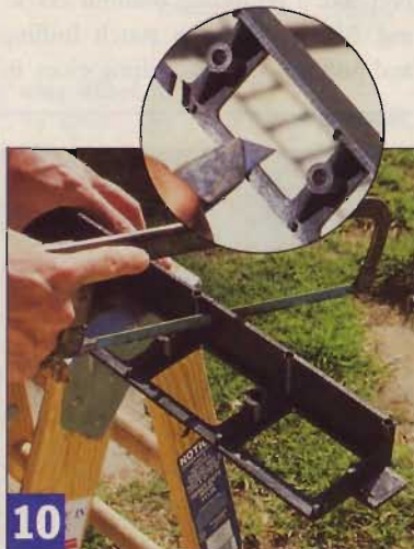
10 Cutting edging to length is easy with a hack saw. Use a knife to cut the webbing to bend the edging along a curve.
