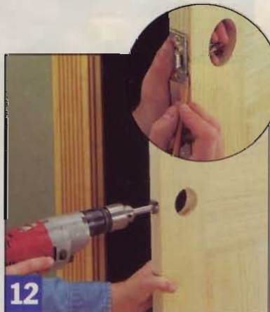
12 For the latch assembly, drill a \frac{1}{8} "-dia. pilot hole first, then follow this guide hole with the 1"-dia. bit. Mark and chisel the mortise for the faceplate.
