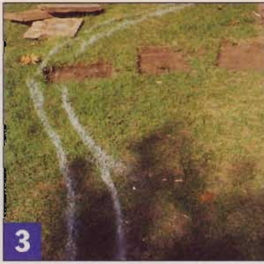
3 Use utility marking paint to outline the walkway once you've developed a fairly clear plan with the hoses or rope.
