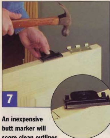
6 Hinge alignment demands precise marking and cutting. Avoid measuring errors by shimming the door in place and marking each hinge location directly.
