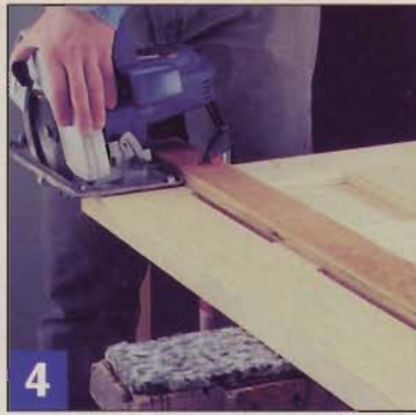
4 Adjustments to the door's width are made along the latch edge. A slight bevel provides clearance for opening and closing, but keeps the tight fit.
