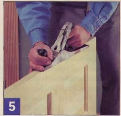
5 Saw marks can be avoided or removed by using a hand plane to bevel the door edge. Planing takes time, but allows you to make fine adjustments.
