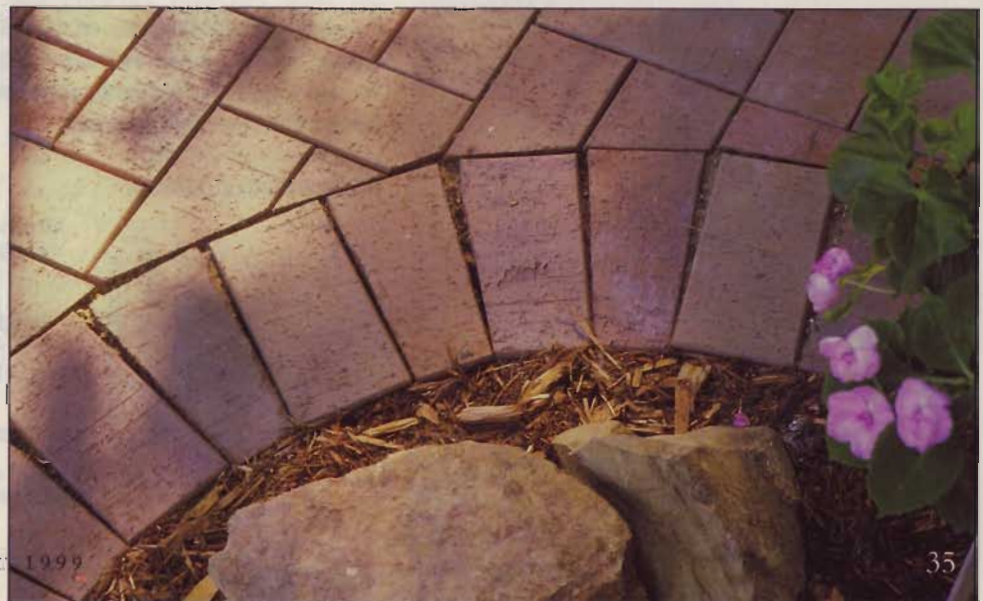
24 When the entire walk is set in place, spread more sand and run the compactor to lock it all together.
