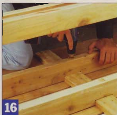
16 With the base aligned over the inverted tabletop, drill 3/16"-dia. pilot holes through the upper stretchers. Then drive #8 x 4" screws in place.
