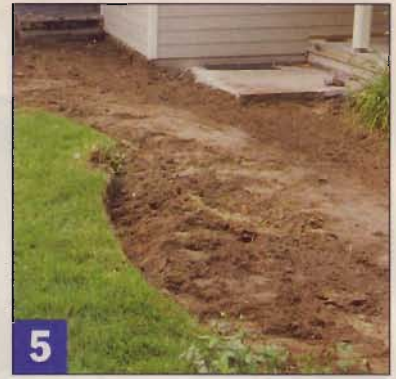
5 Remove sod and soil from the walkway and, for drainage, make sure the path slopes away from the house.
