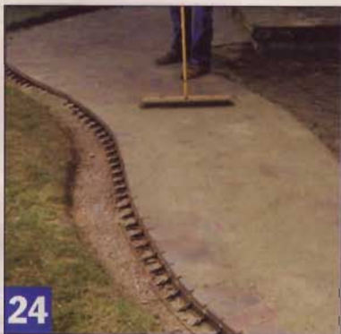
24 When the entire walk is set in place, spread more sand and run the compactor to lock it all together.
