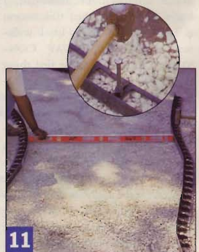
11 The path must be flat and slope away from the house for drainage. Partially drive spikes to hold the edging's shape.
