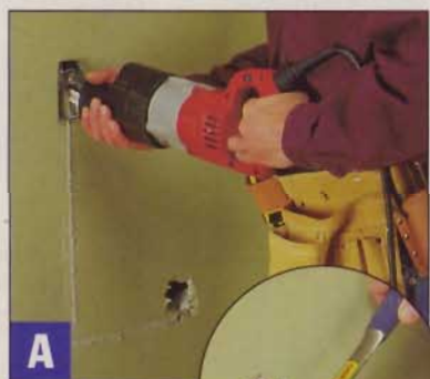
A Punch a small inspection hole to check for wiring and plumbing, then cut a larger hole.
