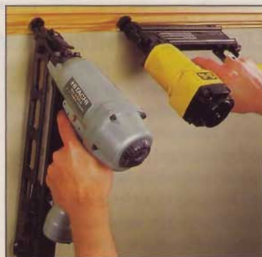
Either type of finish nailer simplifies installing trim, but the angled-magazine (left) allows more angles of approach.
