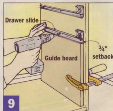
9 A sacrificial guide board positions the slides during installation. Start with the top pair of slides and work your way down, trimming the board as you go.
