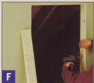
F Jack studs fasten to the existing wall studs and rest on the front sill plate. Install only one side so you have clearance to swing the header into place.
