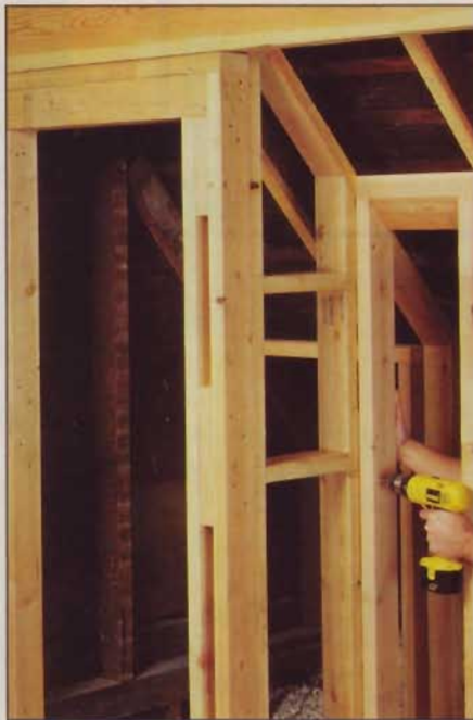
Wall Framing Know-How – 32
