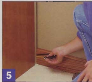
5 Place masking tape along the back edge of each pedestal and use a compass to scribe the pedestal to the wall and base molding.
