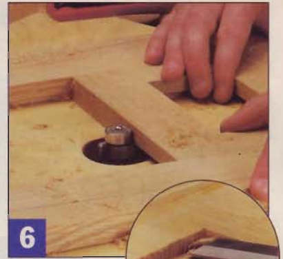
6 Rabbet the glass panel openings at the router table, then square up the corners with a chisel.
