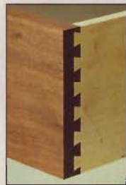
Because the sockets are cut just partway through the pin board, half-blind dovetails are only visible on one side.
