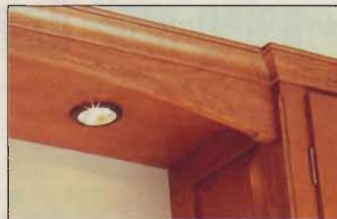
Puck-style xenon lights and cove molding add finishing touches.
