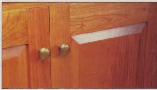
My shop-built cabinets feature 3/8" inset, solid cherry raised panel doors with wide rails. These features weren't available in stock cabinetry.
