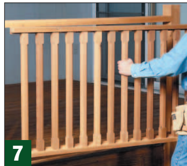
7 With the baluster section assembled, slide it into place. Put the stringer's "lip" toward the interior of the deck.
